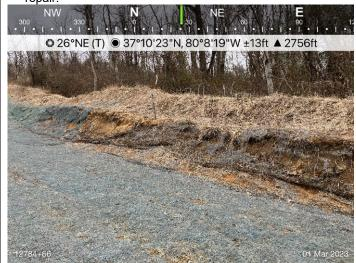
■ Figure 2: Sta 12779 erosion control matting requires repair.
