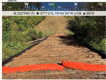
Figure 2: Designated crossing S-G18, ESC controls were in place.
