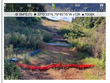
Figure 3: Designated crossing S-G22, ESC controls were in place.
