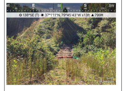
Figure 4: Designated crossing S-G17, ESC controls were in place.
