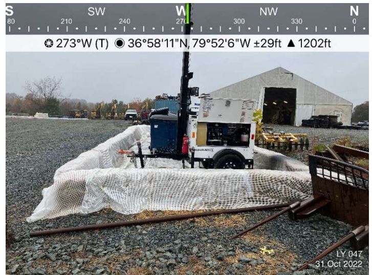
Figure 4: Pollution prevention controls in place and functioning at LY047.
