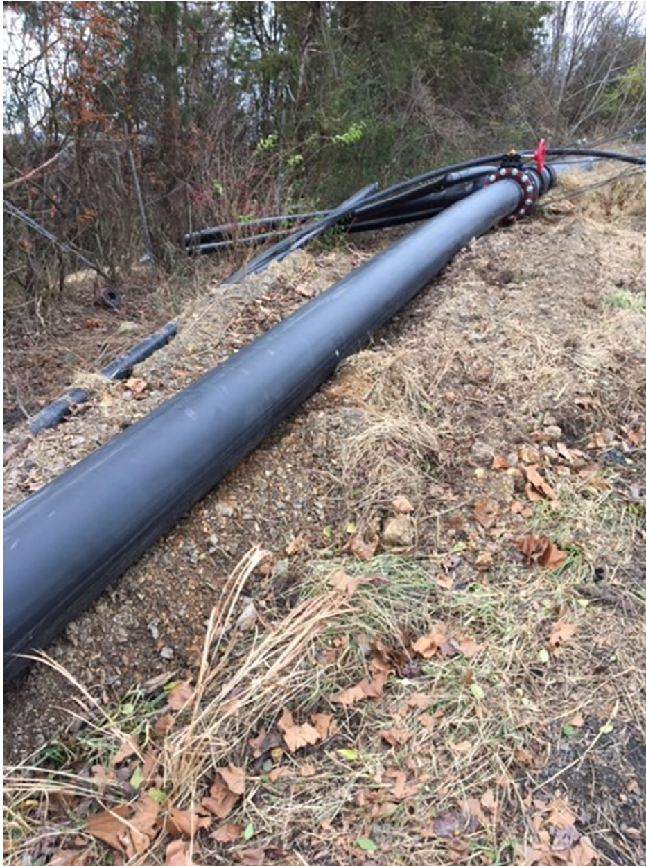
View of 12-inch LFG header tie-in to existing LFG System and 12-inch LFG isolation valve.
