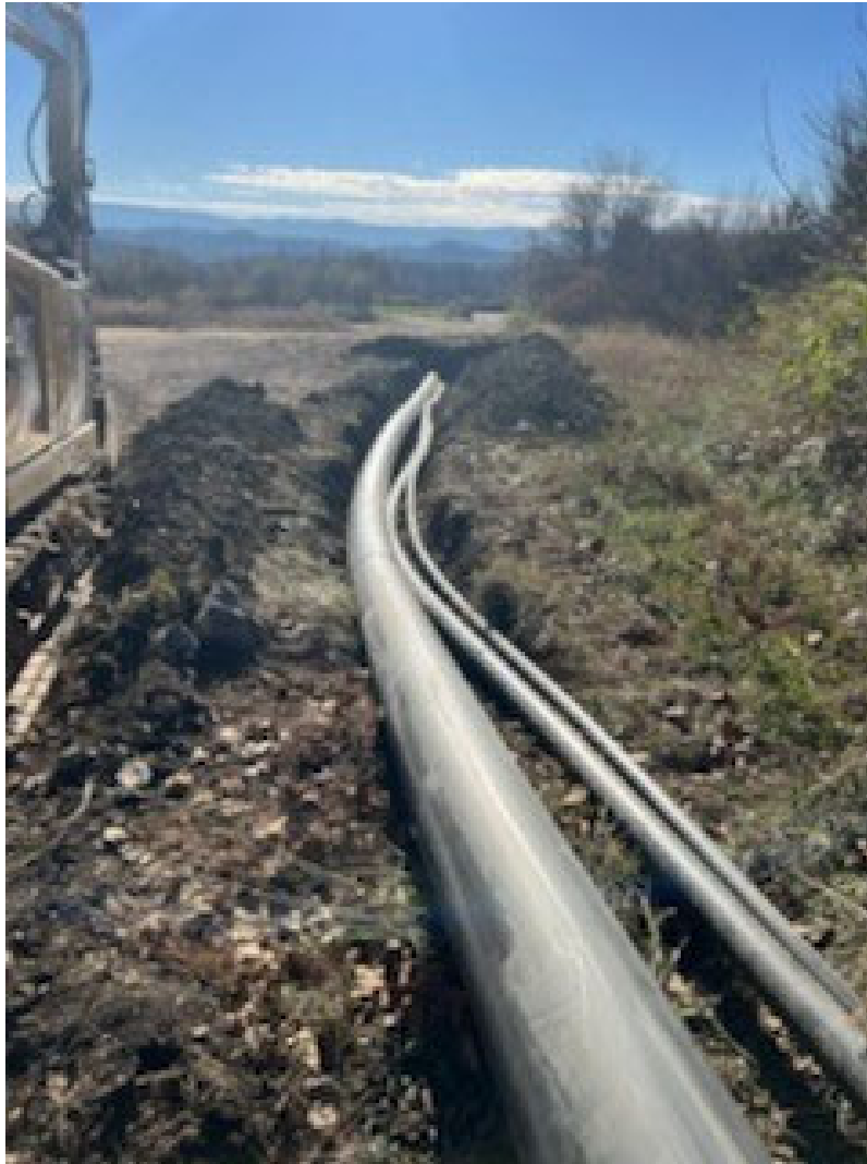
View of 12" LFG header, 2" airline, and 4" forcemain in common trench coming off the existing LFG header tie-in location. Camera facing south.
