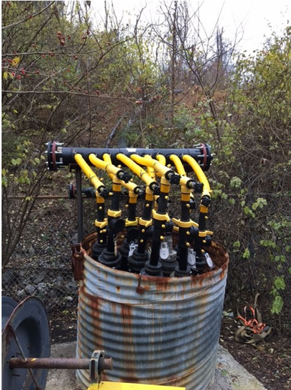
View of south leachate cleanout manifold and nine cleanout tie-ins to the LFG System.
