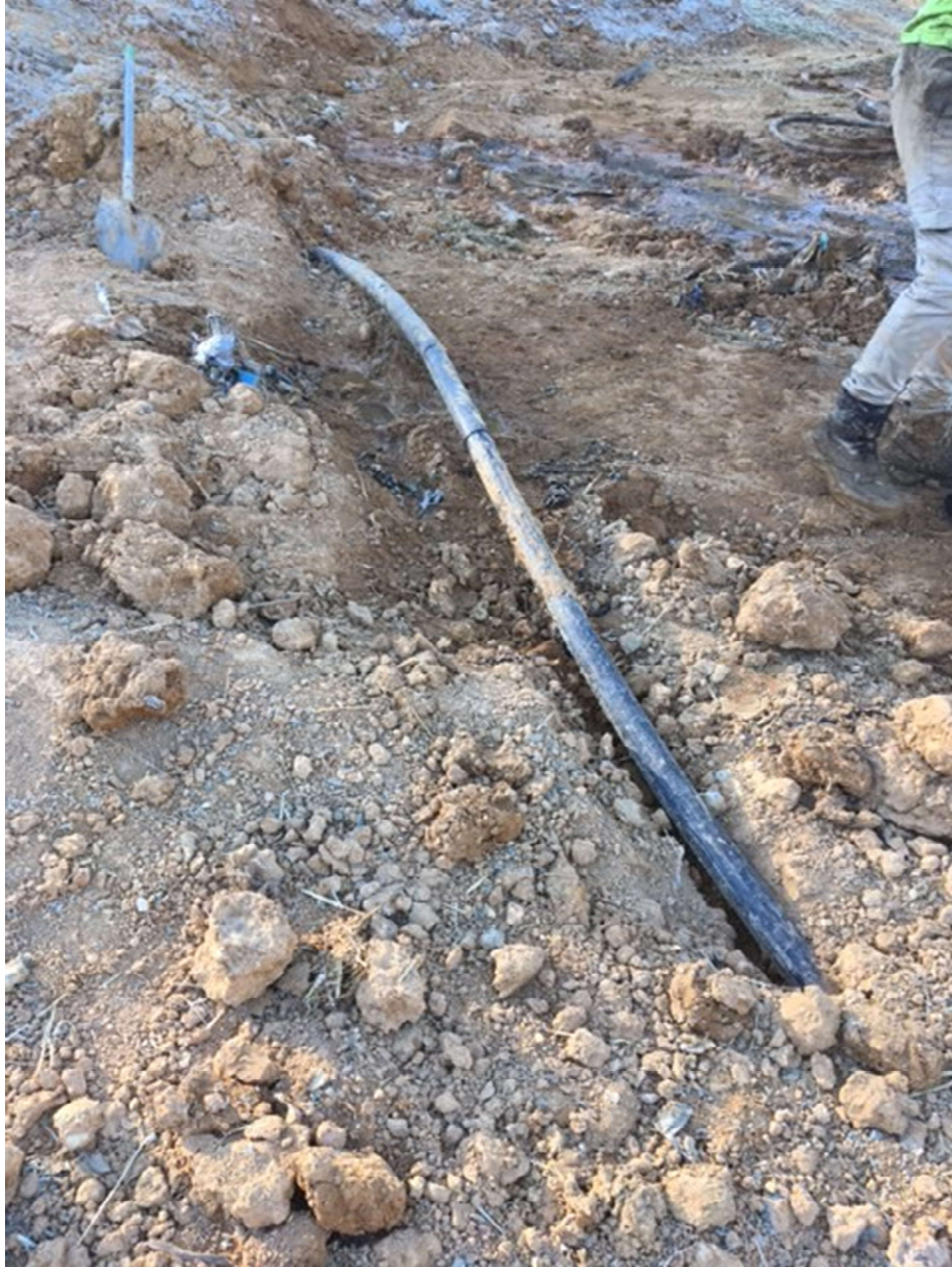
View of airline repair adjacent to temperature probe TP-3.
