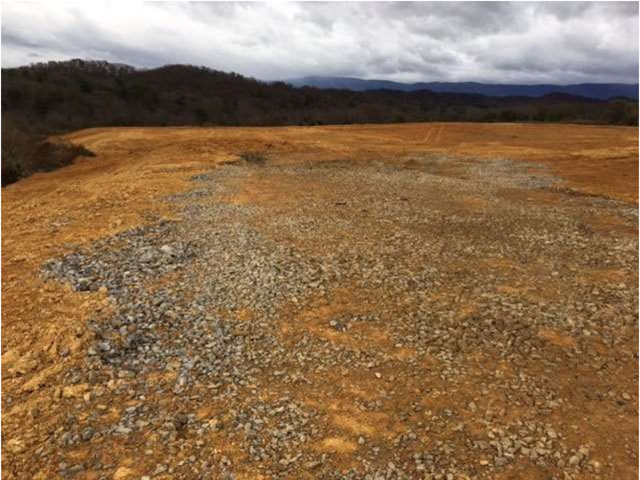
View of Permit No. 498 cover conditions on 11-11-22. Camera facing southeast.
