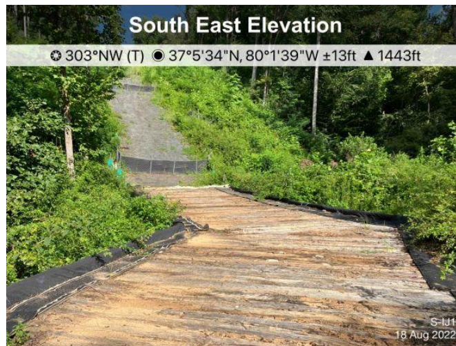
Figure 4: Designated resource W-008, ECD's are in place.
