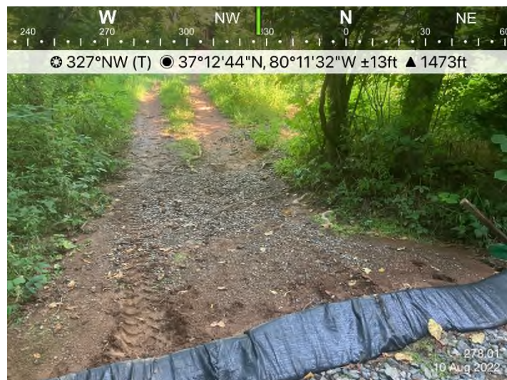
Figure 3: MVP-MN-278.01 – Sediment from denuded driveway moving outside of ROW towards Stream S-EF54.
