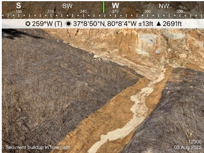
Figure 1: St12900 sediment build up along water bar flow path.
