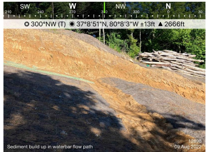
Figure 4: St12898 sediment build up along water bar flow path
