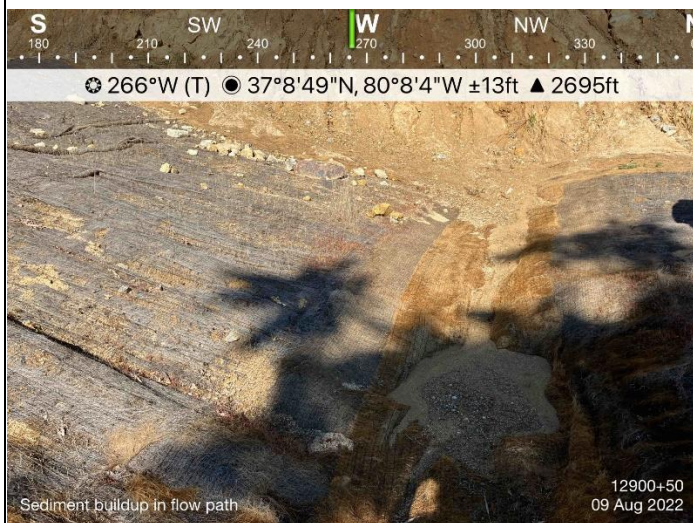
Figure 3: St12900+50 sediment build up along water bar flow path.
