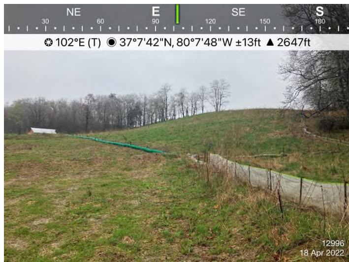
Figure 1: STA 12996+00 – Controls in place and functioning properly.
