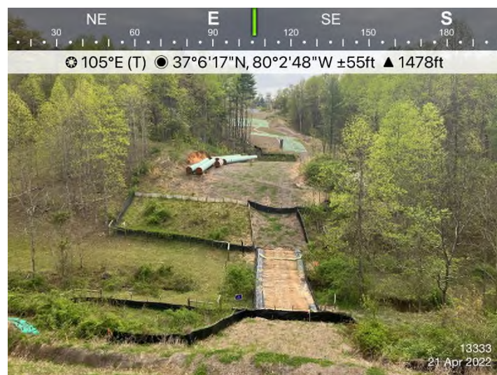
Figure 4: STA 13319+00 – Controls in place and functioning properly.
