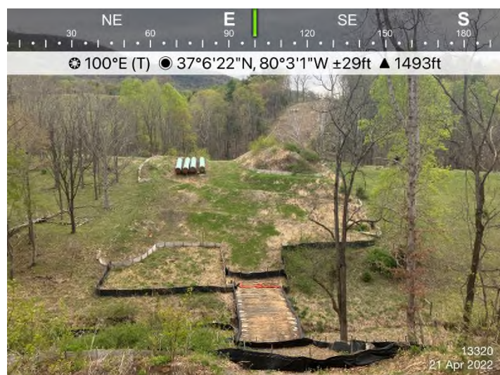
Figure 3: STA 13320+00 – Controls in place and functioning properly.
