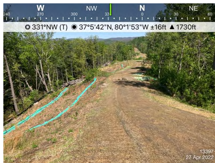
Figure 4: STA 13354+00 – Controls in place and functioning properly.
