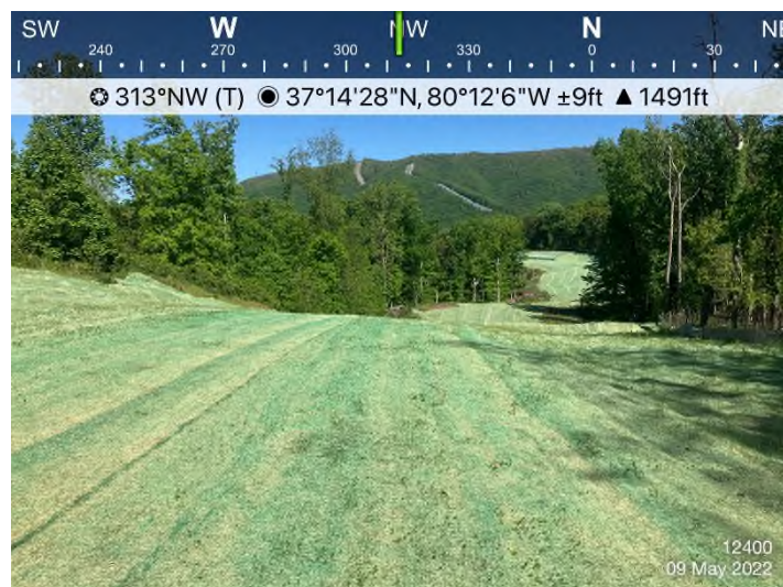
Figure 3: STA 12400+00 – Controls in place and functioning properly. Area stabilized with erosion matting.
