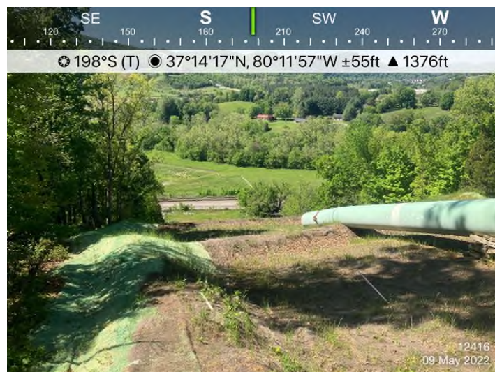
Figure 4: STA 12416+00 – Controls in place and functioning properly. Area stabilized with erosion matting.
