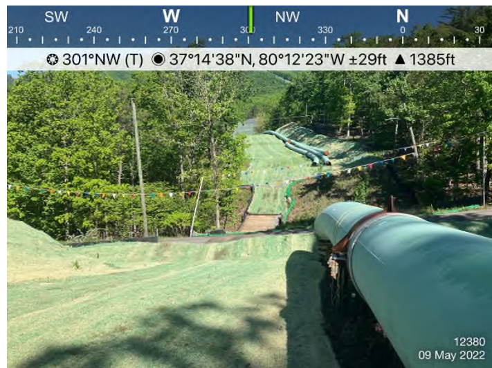
Figure 3: STA 12400+00 – Controls in place and functioning properly. Area stabilized with erosion matting.
