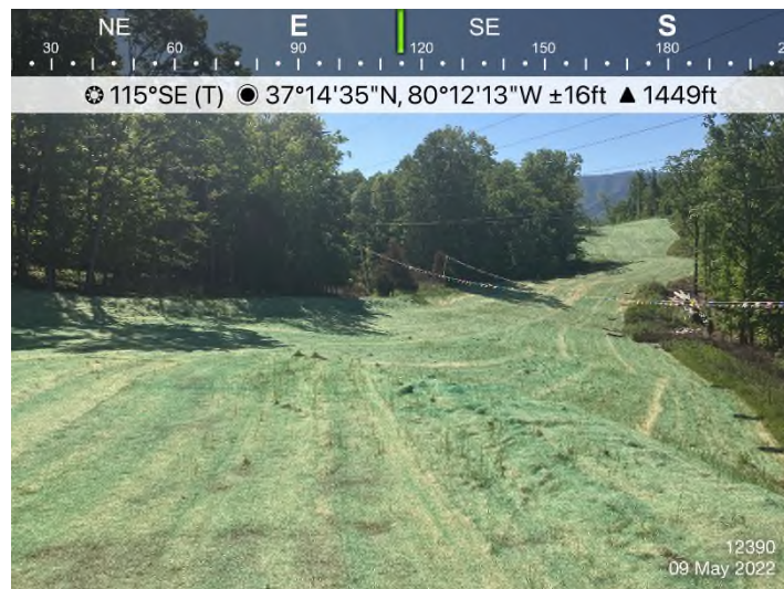
Figure 4: STA 12416+00 – Controls in place and functioning properly. Area stabilized with erosion matting.
