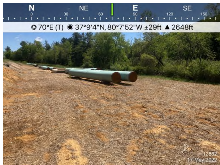
Figure 3: STA 12882+00 – Controls in place and functioning properly. Area stabilized with straw.
