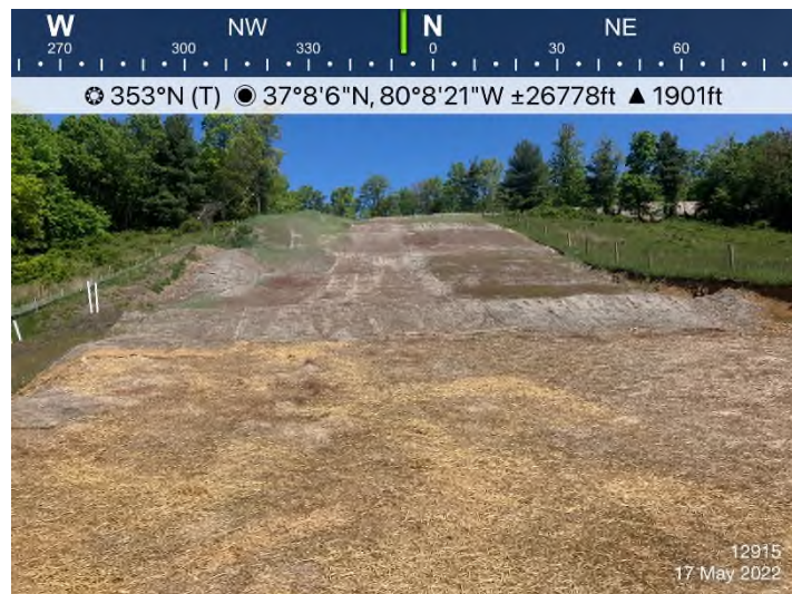
Figure 3: STA 12882+00 – Controls in place and functioning properly. Area stabilized with straw.
