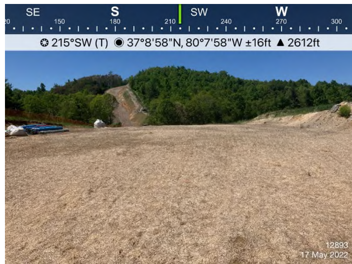
Figure 4: STA 12872+00 – Controls in place and functioning properly. Area stabilized with straw.
