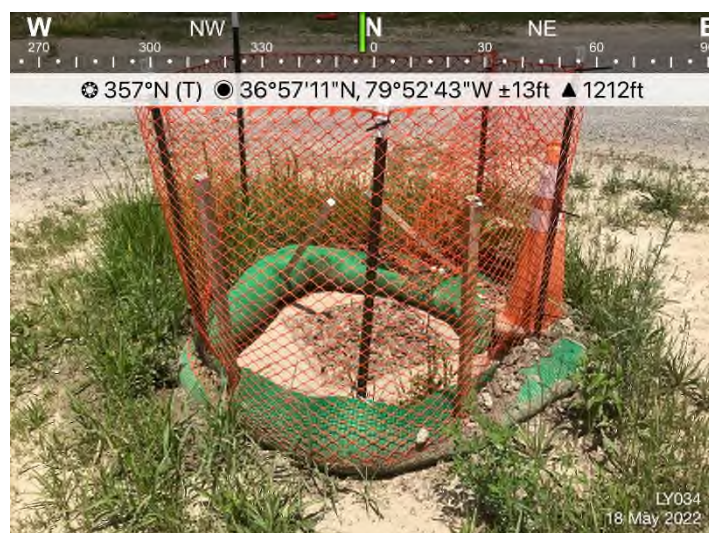
Figure 3: LY 034 – Mulch debris obstructing flow of SW inlet. Maintenance needed.
