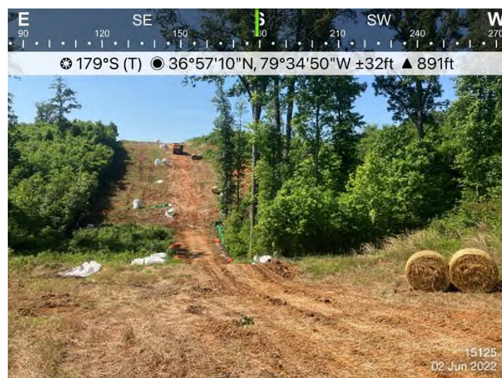
Figure 4: STA 15125+00 – Construction crews actively replacing ECDs and re-stabilizing.
