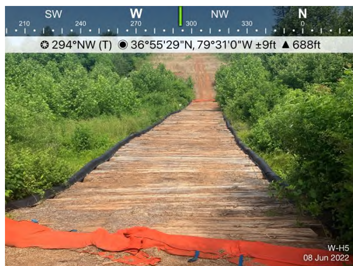
Figure 3: Wetland W-H5 – Controls in place and functioning properly along wetland crossing.
