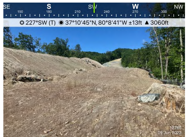
Figure 4: STA 12765+00 – Controls in place and functioning properly. Area stabilized with erosion matting.
