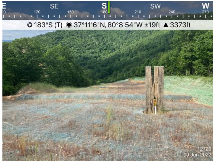
Figure 3: STA 12756+00 – Controls in place and functioning properly. Area stabilized with erosion matting.
