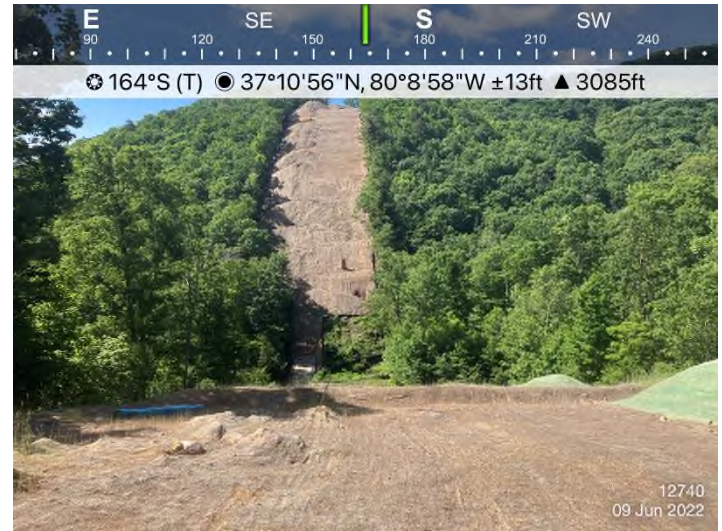
Figure 4: STA 12765+00 – Controls in place and functioning properly. Area stabilized with erosion matting.
