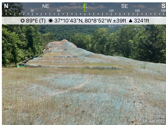
Figure 3: STA 12756+00 – Controls in place and functioning properly. Area stabilized with erosion matting.
