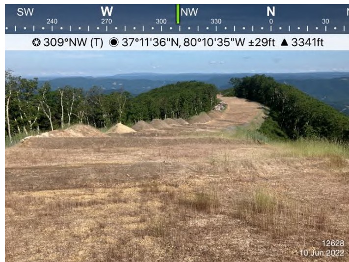
Figure 3: STA 12613+00 – Controls in place and functioning properly. Area stabilized with erosion matting.
