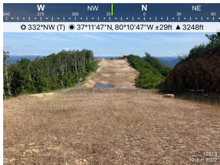
Figure 3: STA 12613+00 – Controls in place and functioning properly. Area stabilized with erosion matting.
