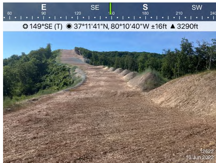
Figure 4: STA 12605+00 – Controls in place and functioning properly. Area stabilized with erosion matting.
