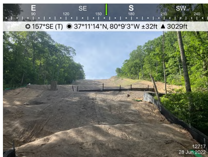
Figure 3: STA 12717+00 – Controls in place and functioning properly. Area stabilized with erosion matting.
