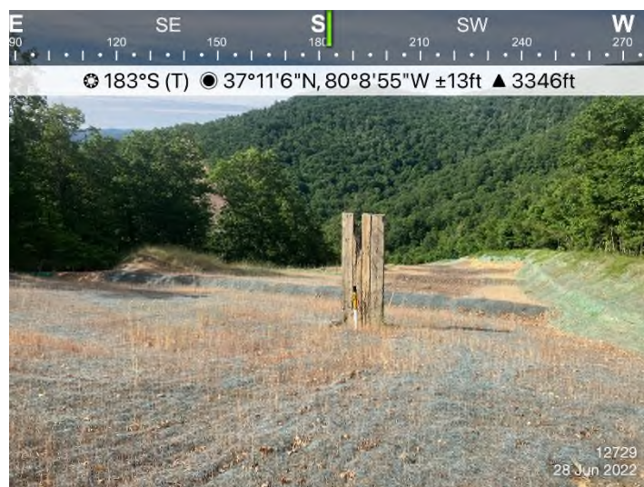
Figure 3: STA 12717+00 – Controls in place and functioning properly. Area stabilized with erosion matting.
