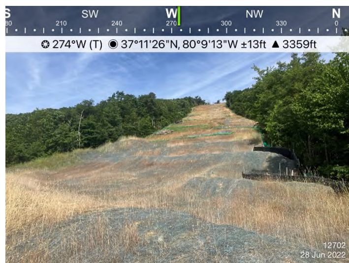
Figure 4: STA 12702+00 – Controls in place and functioning properly. Area stabilized with erosion matting.
