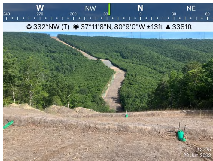
Figure 4: STA 12702+00 – Controls in place and functioning properly. Area stabilized with erosion matting.
