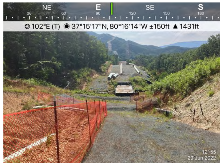
Figure 4: STA 12155+00 – Controls in place and functioning properly. Area stabilized with erosion matting.
