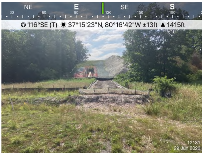
Figure 3: STA 12131+00 – Controls in place and functioning properly. Area stabilized with erosion matting.
