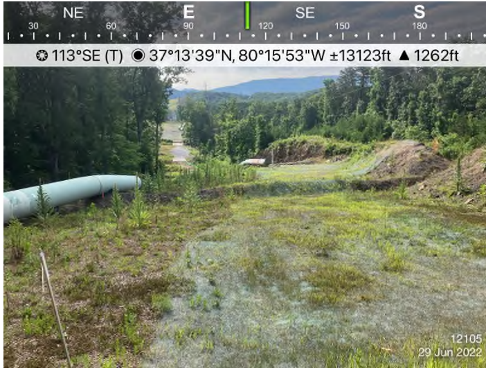
Figure 3: STA 12131+00 – Controls in place and functioning properly. Area stabilized with erosion matting.
