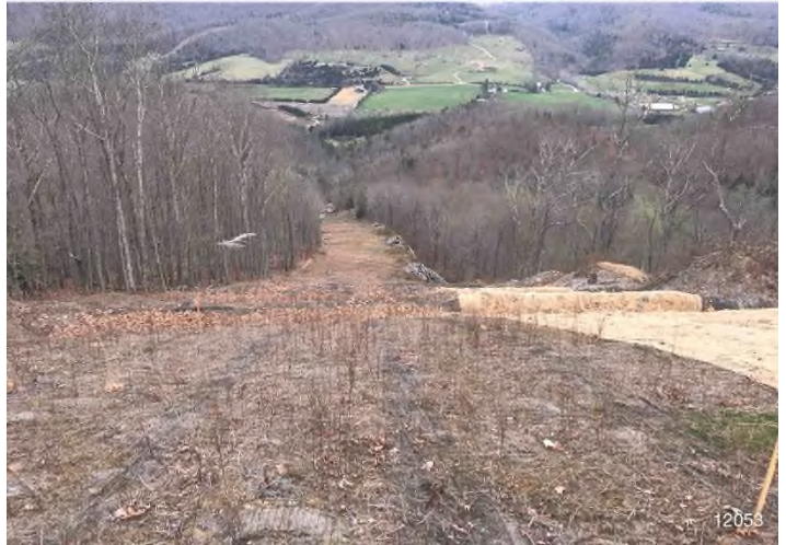
Figure 4: STA 12028+00 – Controls in place and functioning properly.
