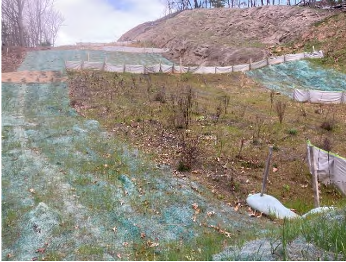
Figure 3: STA 12504+00 – Controls in place and functioning properly. Area stabilized with erosion control matting.
