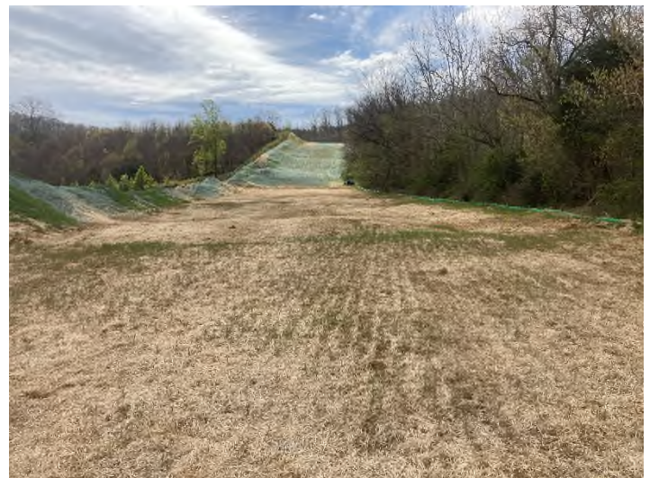
Figure 4: STA 12471+00 – Controls in place and functioning properly. Area stabilized with straw.
