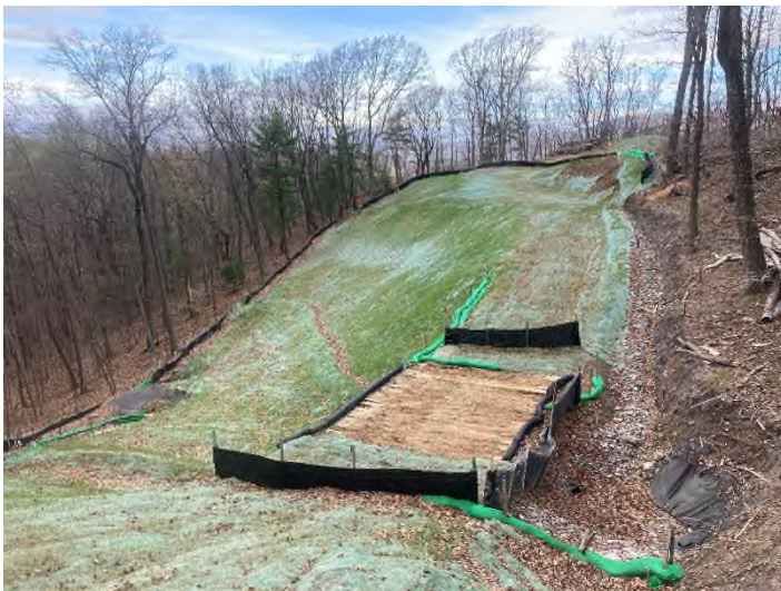
Figure 3: STA 12504+00 – Controls in place and functioning properly. Area stabilized with erosion control matting.
