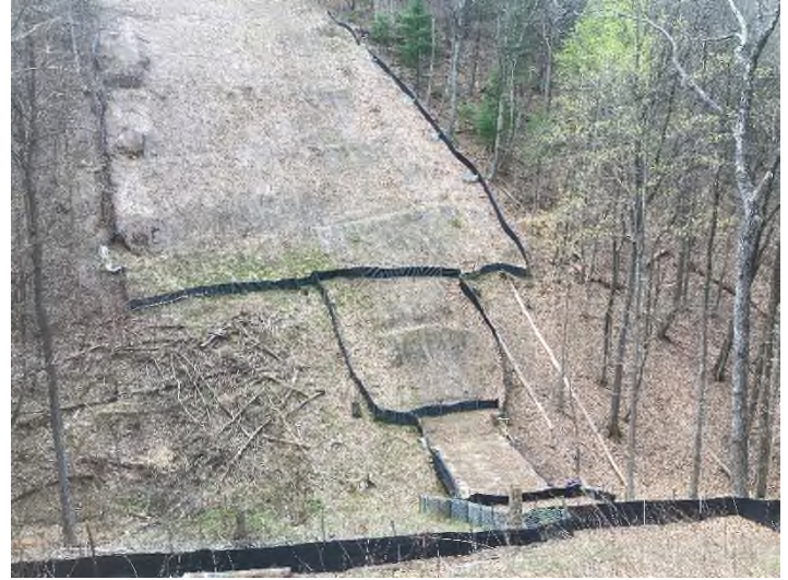
Figure 4: STA 12471+00 – Controls in place and functioning properly. Area stabilized with straw.
