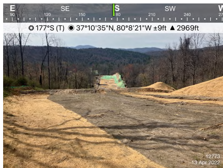
Figure 3: STA 12773+00 – Controls in place and functioning properly. Area stabilized with erosion control matting.
