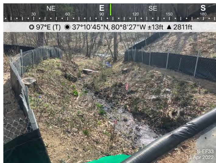
Figure 4: STA 12763+00 – Controls in place and functioning properly. Area stabilized with erosion control matting.
