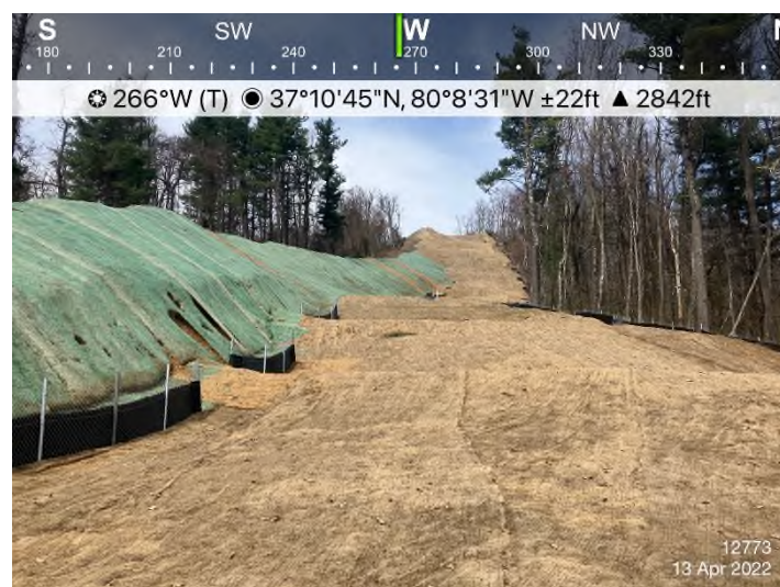
Figure 4: STA 12763+00 – Controls in place and functioning properly. Area stabilized with erosion control matting.
