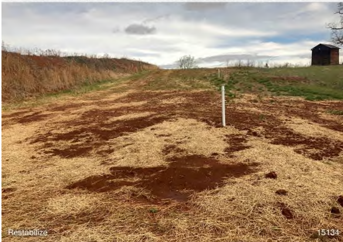
Figure 3: STA 15134+00 – Re-stabilization needed.
