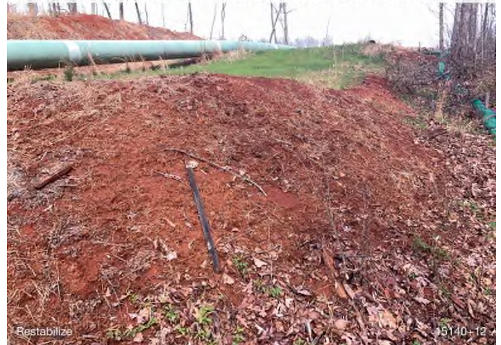
Figure 4: STA 15140+12 – Re-stabilization needed.
