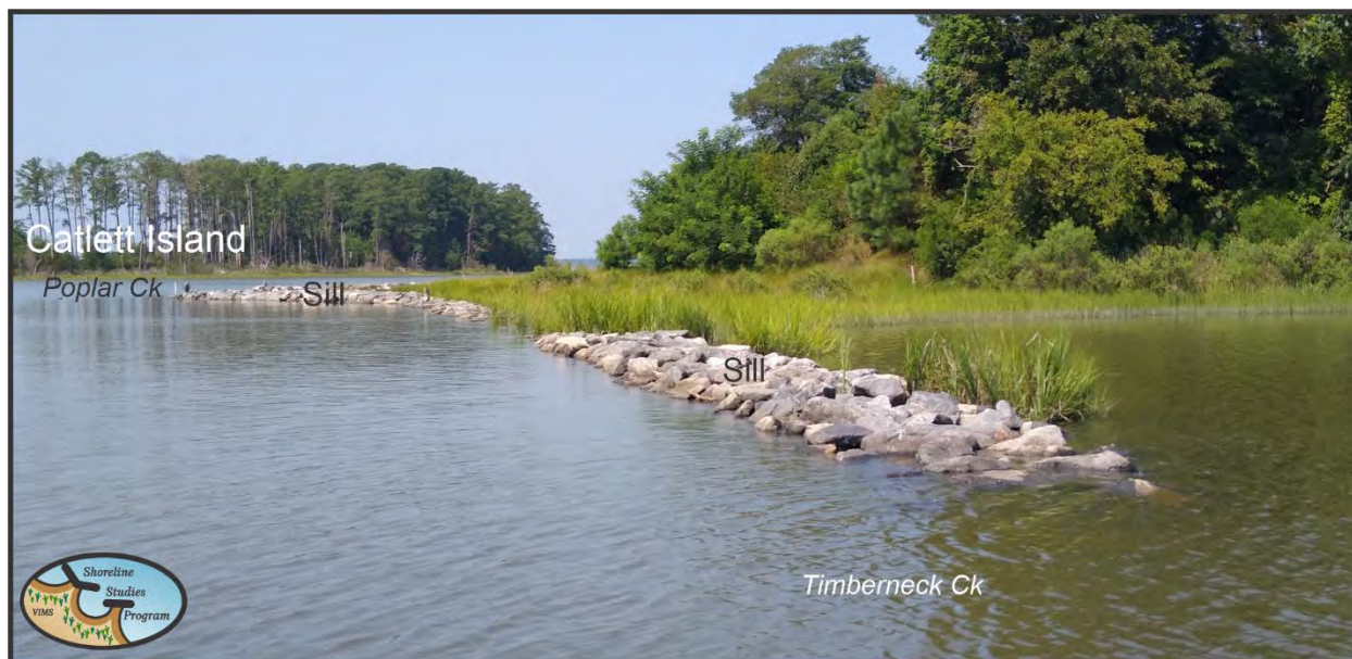
Figure 6. Sill constructed at the southeastern tip of the park on Timberneck Creek in 2011. Photo date 24 Aug 2021. Lat/long location: 37.294578°, -76.534841°
