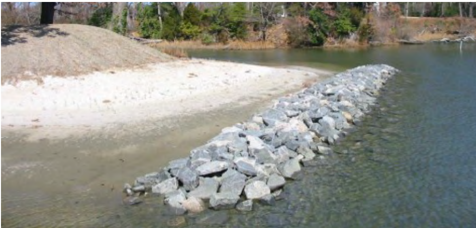
Photo taken 4 Mar 2011 1258 New sill, placed sand nourishment, marsh grass planted, fill placed over bank instead of grading it. Photo credit: VMRC Project Report dated 4 Sep 2009
