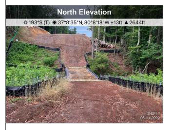
Figure 4: ATWS 954, remains dormant and ECD's are in place.
