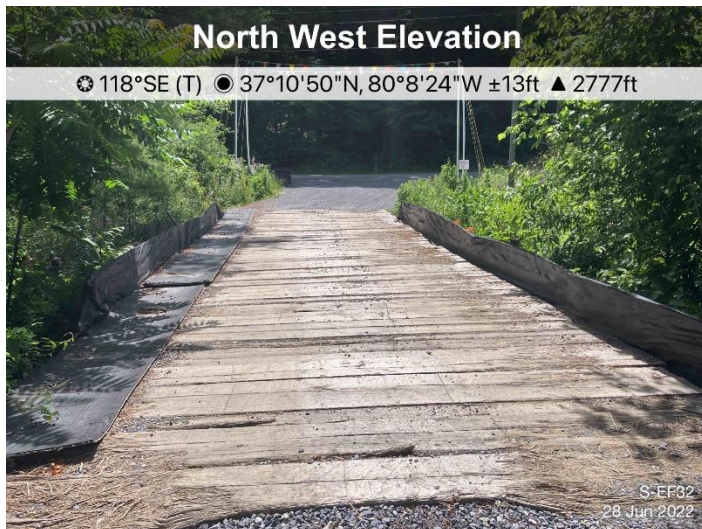
Figure 3: Designated crossing S-EF32, ECD's are in place.
