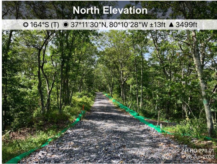
Figure 1: AR RO 279.01 ECD's are in place.
