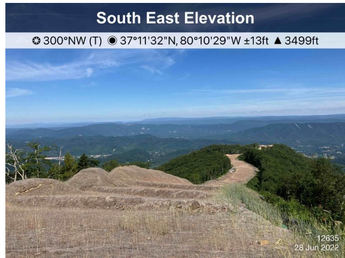
Figure 4: St12635, ECD's and stabilization are in place.
