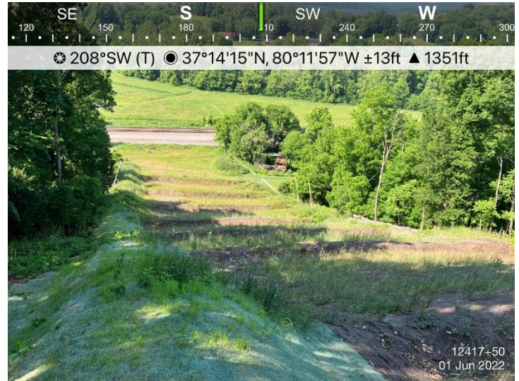
Figure 2: St 12417+50, ECD's and stabilization in place.
