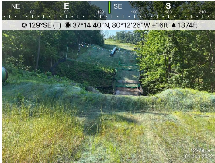
Figure 1: St 12378+84, ECD's and stabilization in place.
