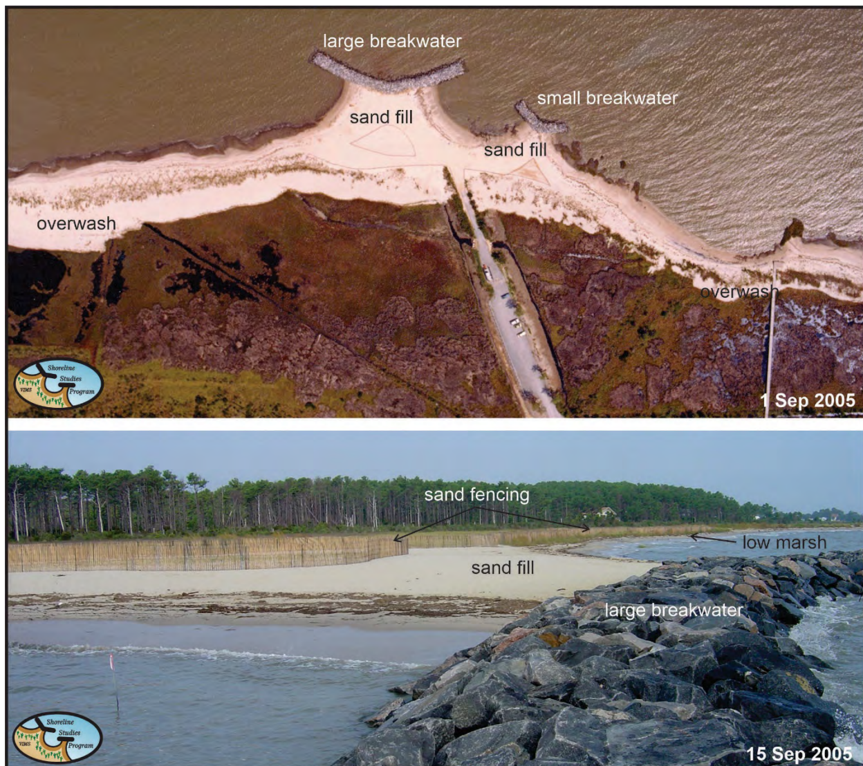
Figure 8-7. Haven Beach in 2005 just after the construction of the shore protection system. Sand fill was placed behind the structures and sand fencing was installed to help maintain the sand in the system. Photo credit: Shoreline Studies Program, VIMS.
