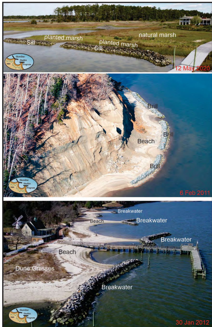
Figure 4-1. Top shows a sill with planted marsh at Captain Sinclair's Recreational Area, Gloucester, VA; Middle shows a brill at Westmoreland State Park; and Bottom shows headland breakwaters and beach fill at Yorktown, VA. Photo credit: Shoreline Studies Program, VIMS.
