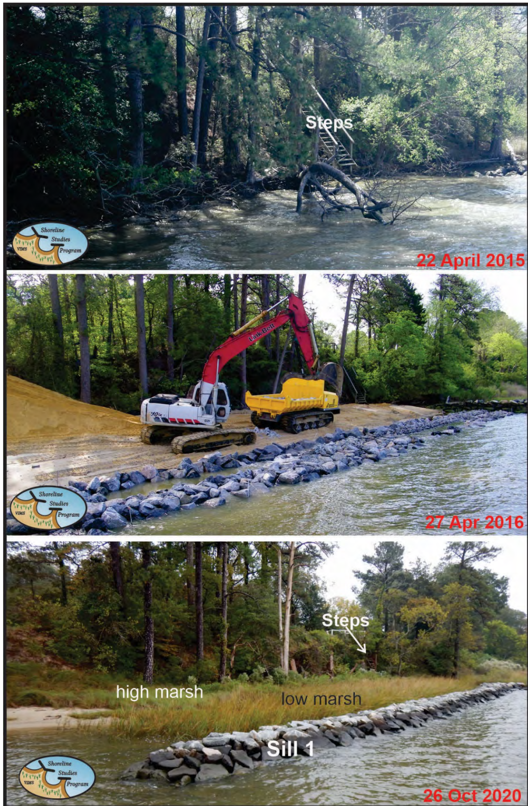
Figure 7-12. Pre-project shoreline showing an eroding bank with fallen trees (top); During construction of Sill 1 (middle); and Sill 1 about 4.5 years after construction showing a lush marsh (bottom). Photo credit: Shoreline Studies Program, VIMS.
