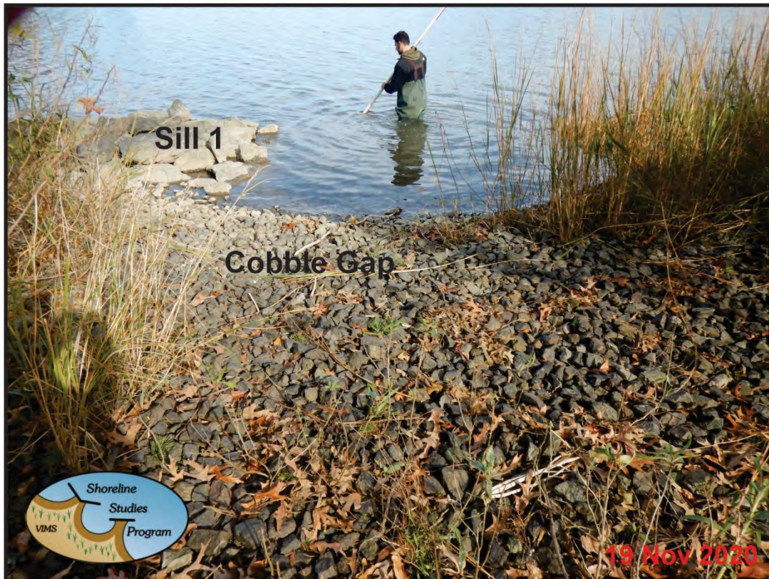
Figure 9-18. Ground photo of the site showing the cobble sill gap. Photo credit: VIMS, Shoreline Studies Program.
