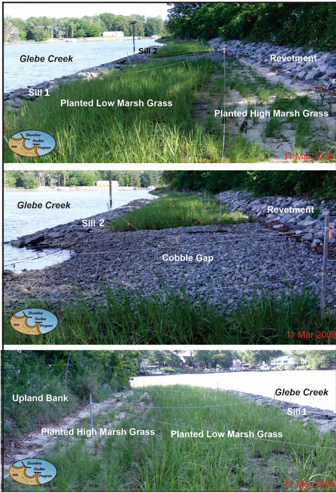
Figure 9-11. Hull Springs Farm living shoreline after about 1 year. The elements were constructed as designed, and the low marsh has filled in well. Photo credit: Shoreline Studies Program, VIMS.
