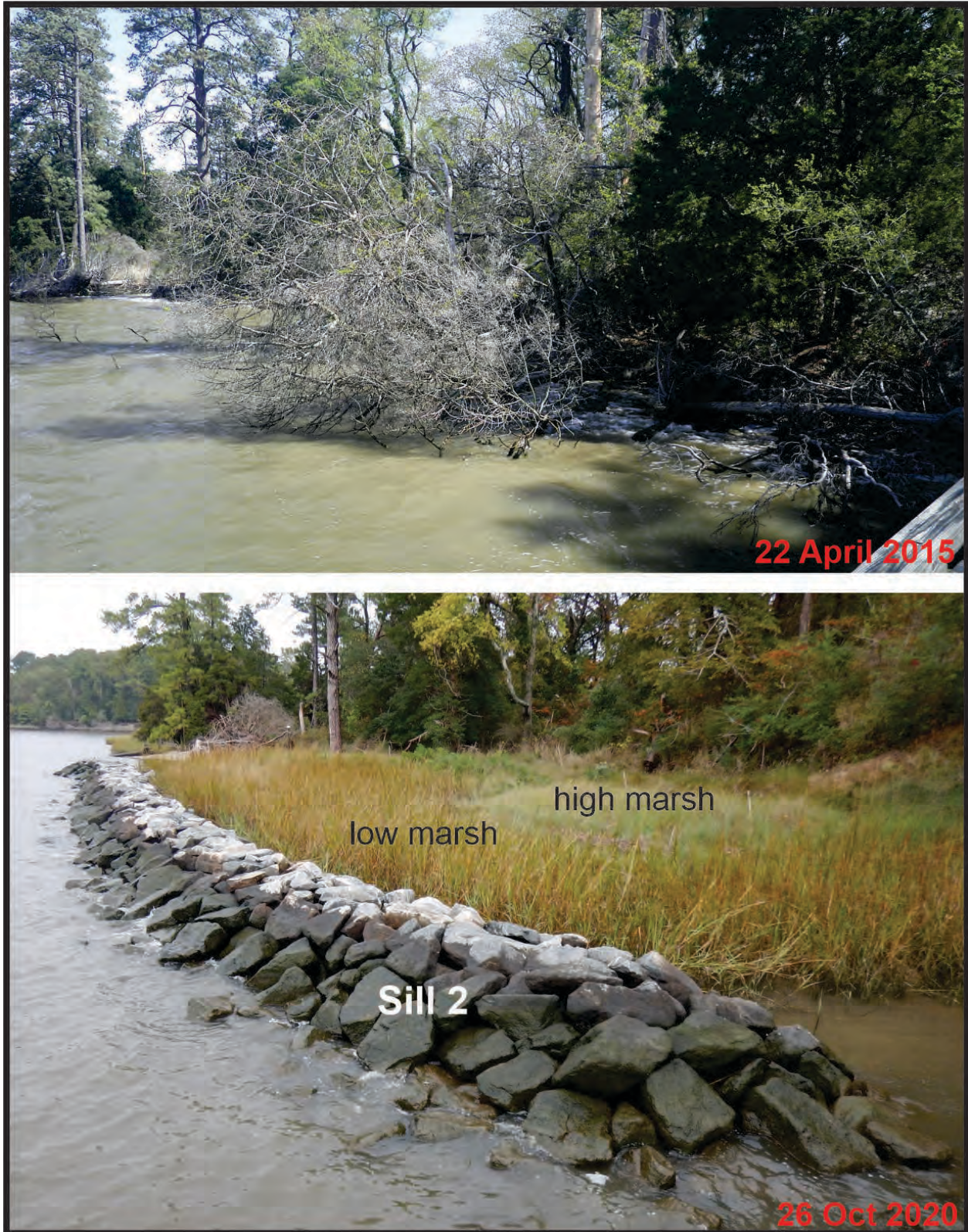
Figure 7-11. Pre-project shoreline showing an eroding bank with fallen trees (top); and Sill 2 about 4.5 years after construction showing a lush marsh (bottom). Photo credit: Shoreline Studies Program, VIMS.
