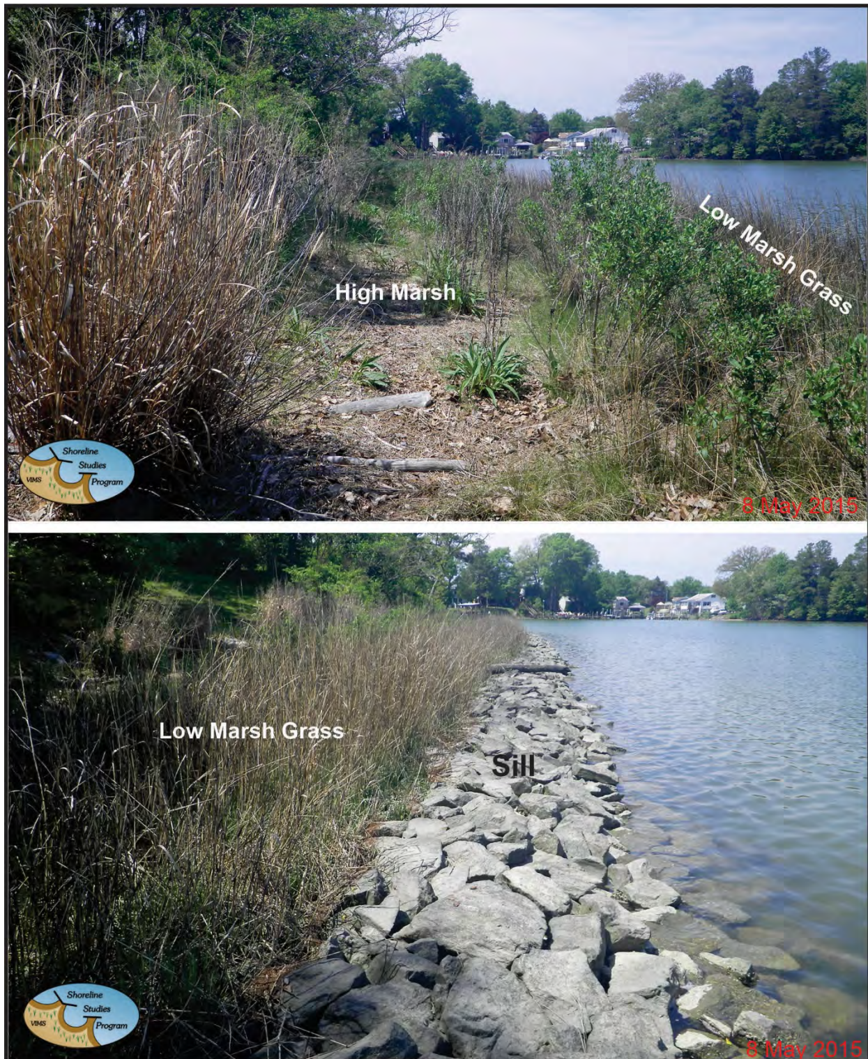
Figure 9-13. Hull Springs Farm about 6 years after construction. Top: The backshore where the upper marsh should be does not have as much grass vegetation as the low marsh. Bottom: The low marsh is doing well behind sill 1. Photo credit: Shoreline Studies Program, VIMS.
