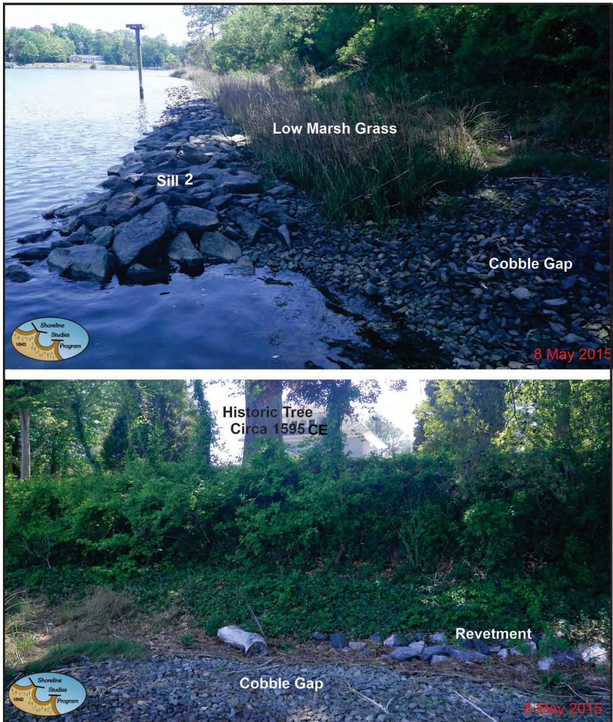
Figure 9-12. Hull Springs Farm about 6 years after construction. Top: Sill 2 has lush low marsh behind the structure, but the high marsh is not as vegetated. Bottom: The bank has slumped over the revetment. The sediment is vegetated which adds additional stability to the bank to protect the historic tree. Photo credit: Shoreline Studies Program, VIMS.
