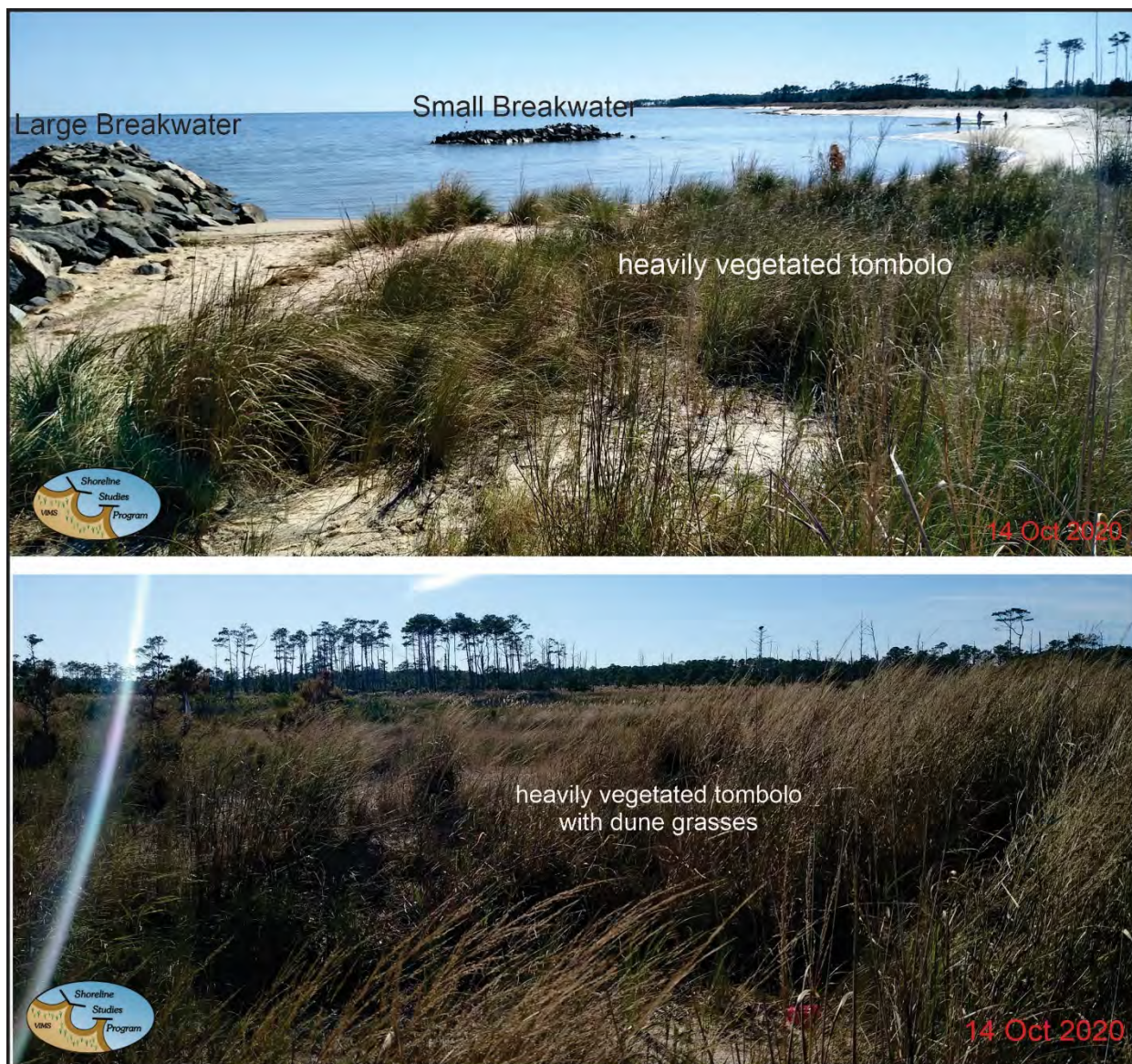
Figure 8-14. Ground photos showing the tombolo behind the large breakwater. Photo credit: Shoreline Studies Program, VIMS
