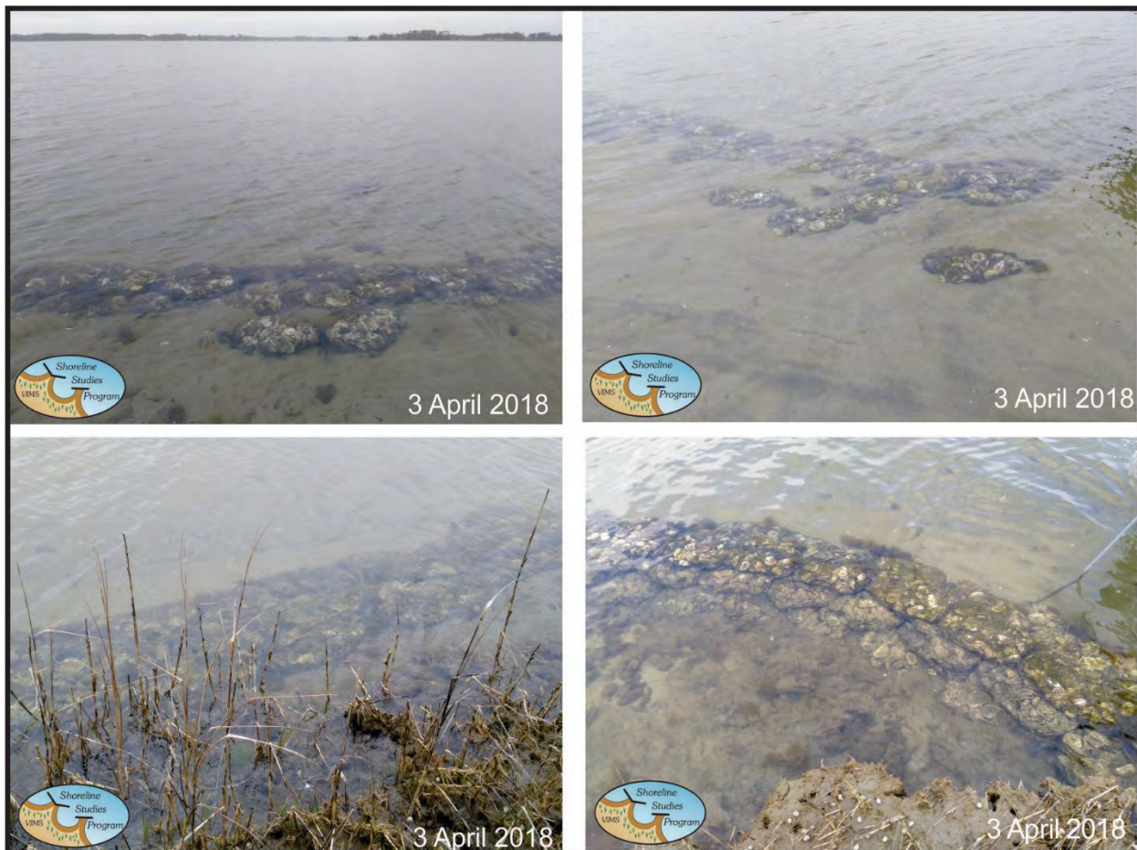
Figure 4-3. Captain Sinclair's Recreational Area oyster bag sill. The three-bag sill (top) that was placed on the southwest-facing shoreline has not been as stable. The top bag of some sections were rolled toward the shoreline. The six-bag sill (bottom) on the point and the southeast-facing shoreline has remained intact. From Milligan et al. (2018).
