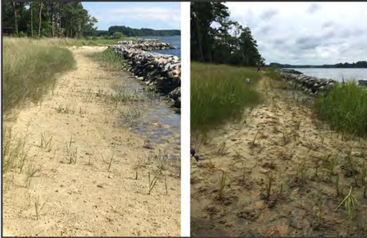
Figure 5-8. Photos showing a bare spot behind the sill (left) in May 2017, and the grasses replanted in July 2017 (right).
