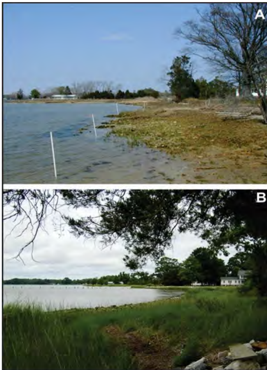
Figure 4-4. Hollerith marsh toe revetment/sill site A) before project with eroding fringing marsh in winter and B) after construction.
