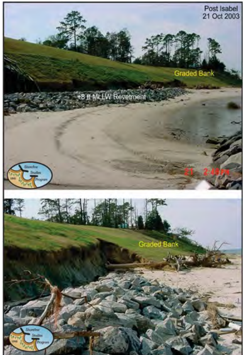
Figure 3-11. Revetment on the James River that was overtopped by storm surge and waves during Hurricane Isabel. Photo dates 21 October 2003.
