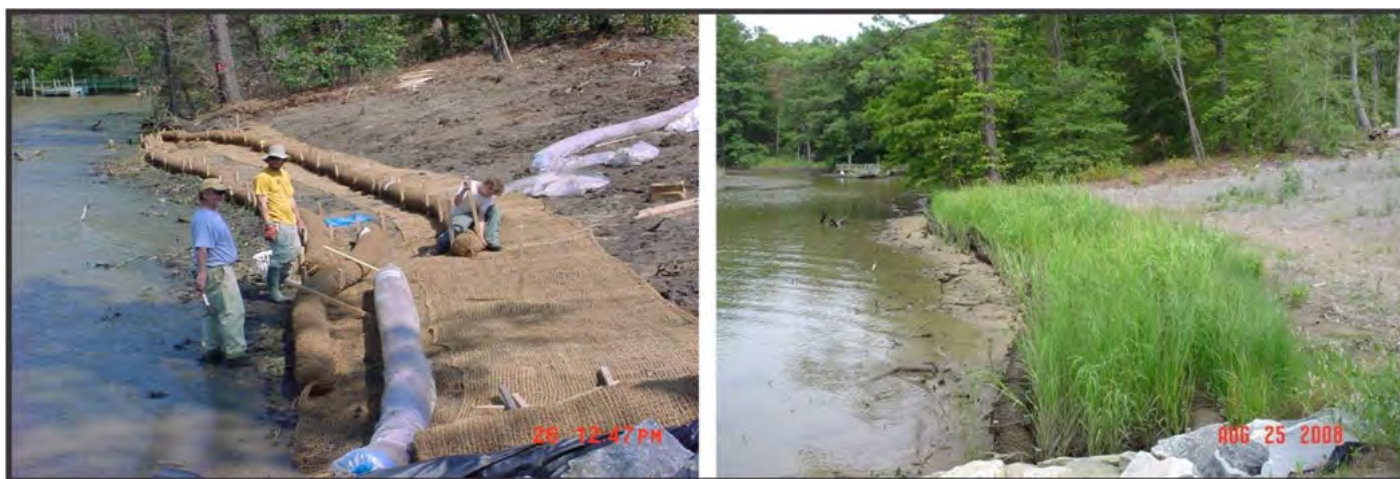
Figure 3-3. Coir logs and mats placed at toe of a graded bank for temporary stabilization while planted tidal marsh and riparian buffer become established. Photos by P. Menichino.
