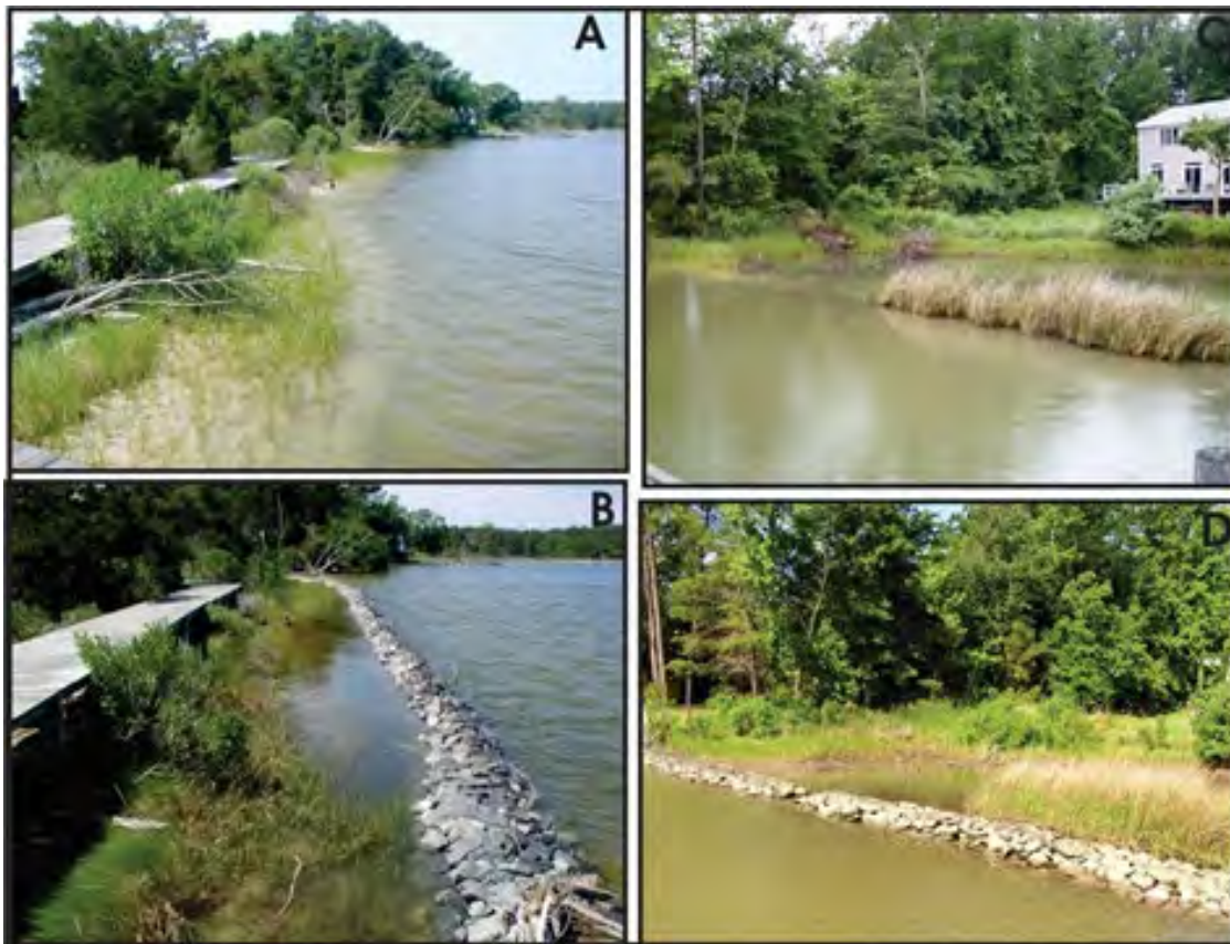
Figure 3-6. Photos showing marsh toe revetments A) before and B) after a project on Cranes Creek in Northumberland County and C) before and D) after a project on Mosquito Creek in Lancaster County, Virginia.
