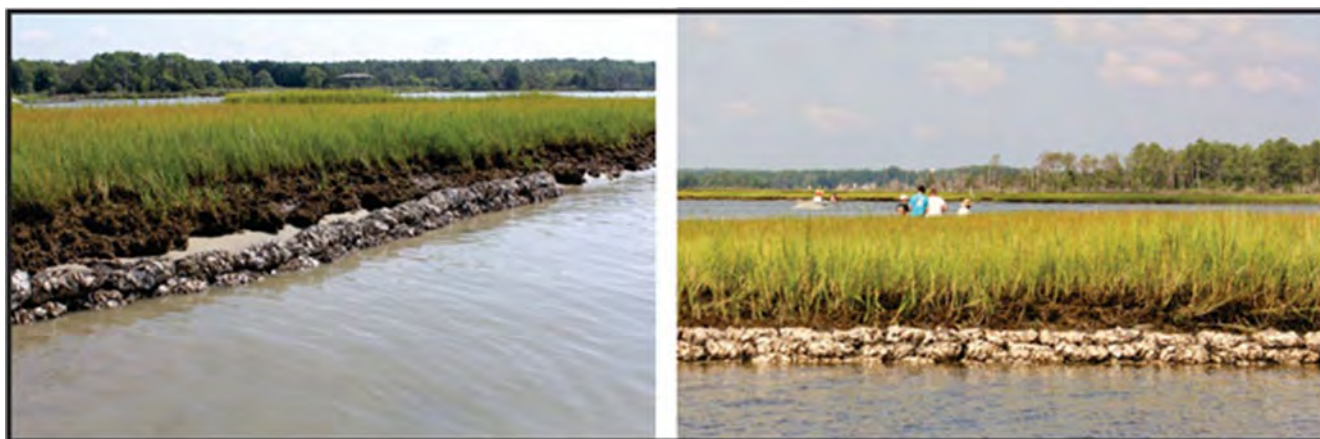
Figure 4-2. Construction of the 3-bag sill (left) and 6-bag sill (right) in August 2017. From Milligan et al. (2018). Photo credit: Linda Tjossem
