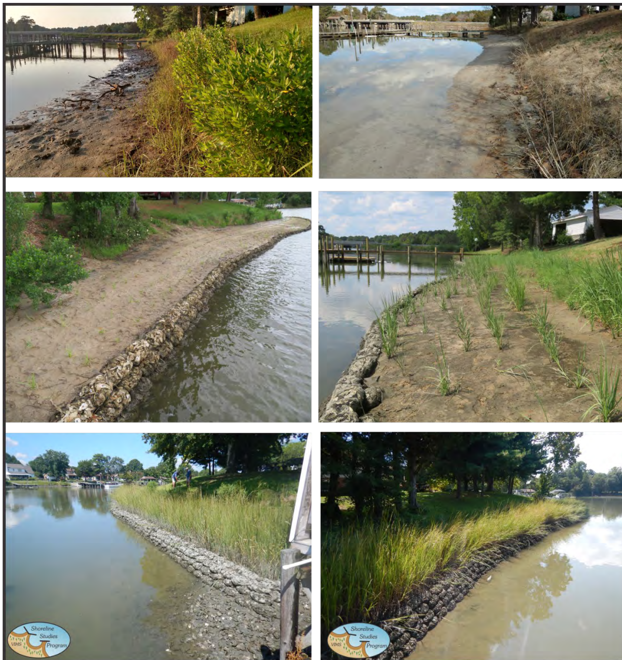
Figure 3-7. An example of the construction of oyster reef bags with sand fill and marsh grasses planted behind the structures. Top left: Shoreline prior to the project on 26 May 2016; Top right: after the sand fill was placed May 2017; Middle left: after bags were placed in May 2017; and Middle Right: after the grass was planted in July 2017. Photo credit: Walter Priest. Bottom right and left: Site about 1.5 years after construction.
