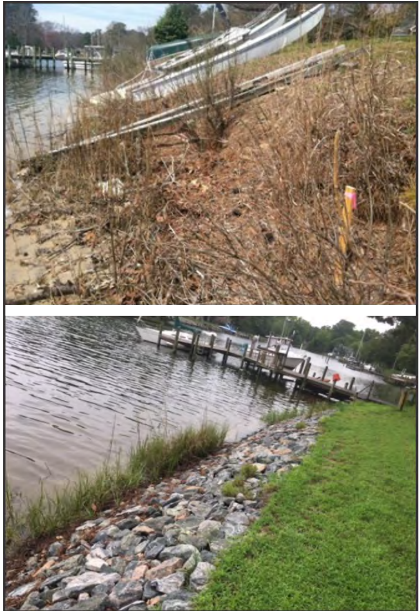
Figure 4-1. The Poole site in 2016 (top) showing the loss of much of the intertidal marsh fringe, and in 2018 (bottom) after the construction of a riprap revetment along the bank above mean high water. Photos from the VMRC permit (#20160366) report.
