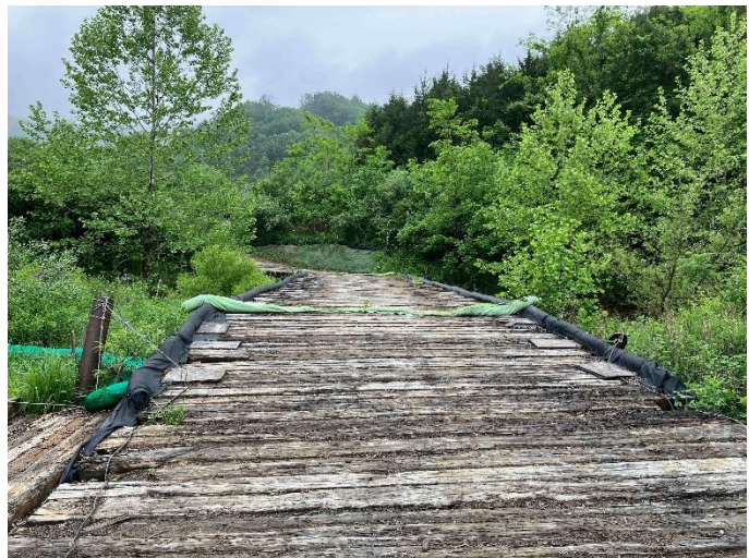
Figure 4: Designated crossing S-G36 on AR MN268, ECD's are in place.
