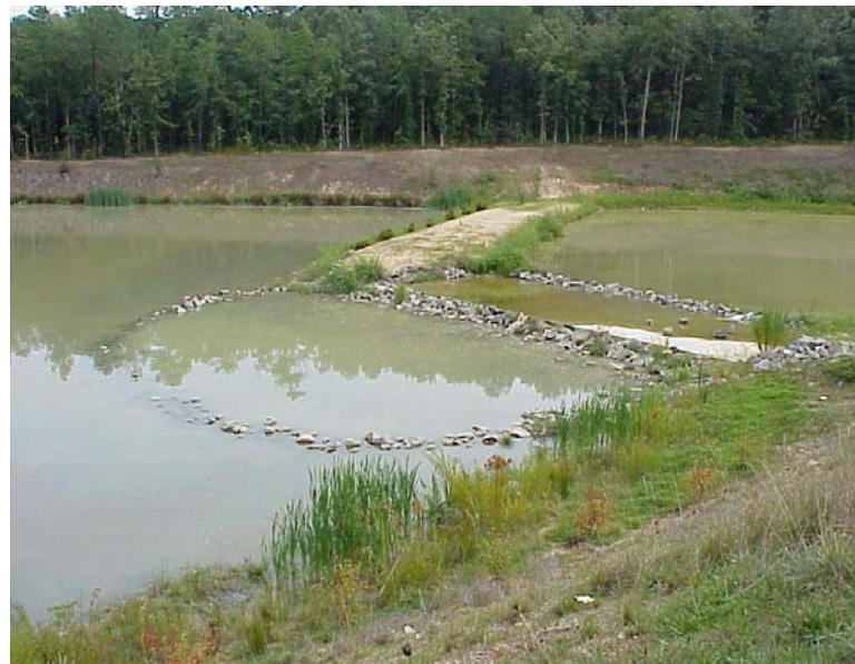
Sediment Forebay constructed with submerged rip-rap weir.
