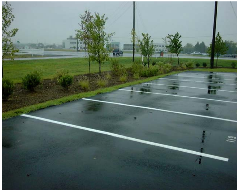
Bioretention Basins in office setting parking lot.
