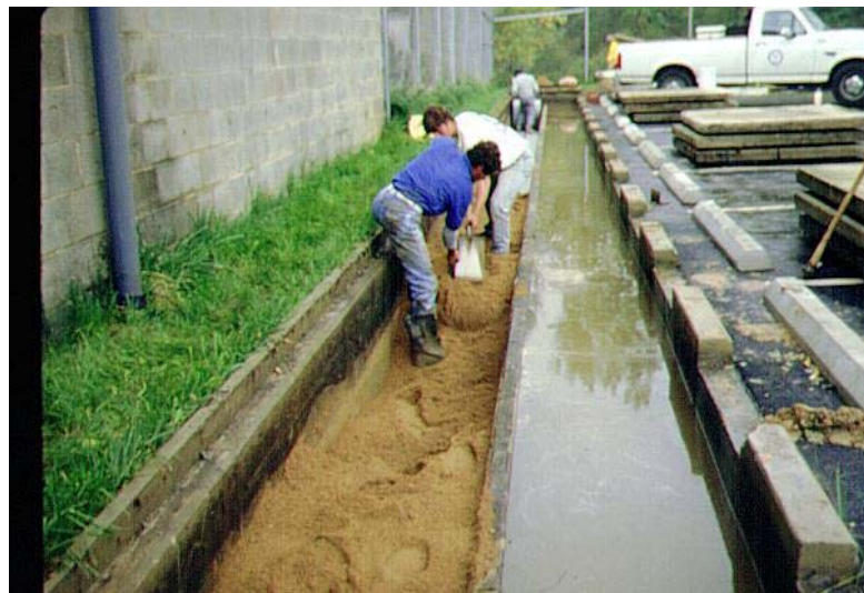
Sand Filter under construction. Note curb cuts for inflow to wet chamber with weir overflow into sand chamber.
