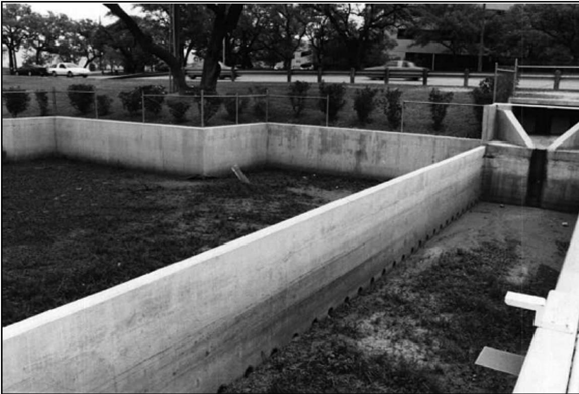
FIGURE 3.12 - 1 Austin Partial Sedimentation Surface Sand Filter
