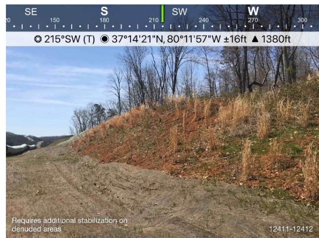
Figure 4: Additional stabilization near stations 12411-12412 required.
