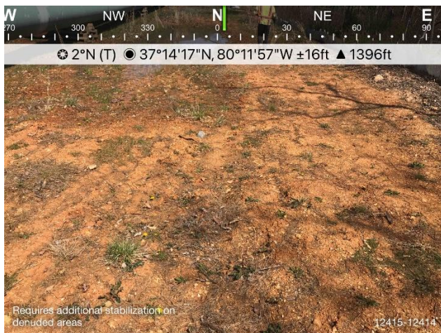
Figure 3: Additional stabilization near stations 12415-12414 required.
