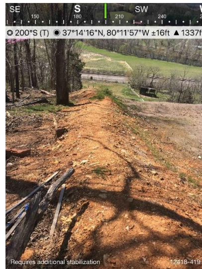
Figure 2: Additional stabilization required near stations 12418-12419
