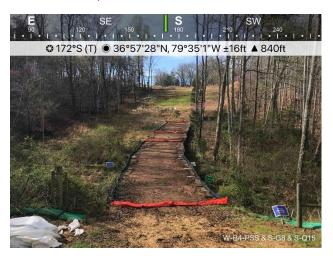
Figure 2: St 15064-15065, stockpile requires additional stabilization.
