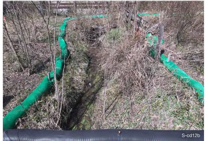
Figure 4: Stream S-CD12b – Controls in place and functioning properly around stream crossing. BRG: 360°N (T) LAT: 37.229833 LON: -80.201264 ±16ft ALT: 1203ft
