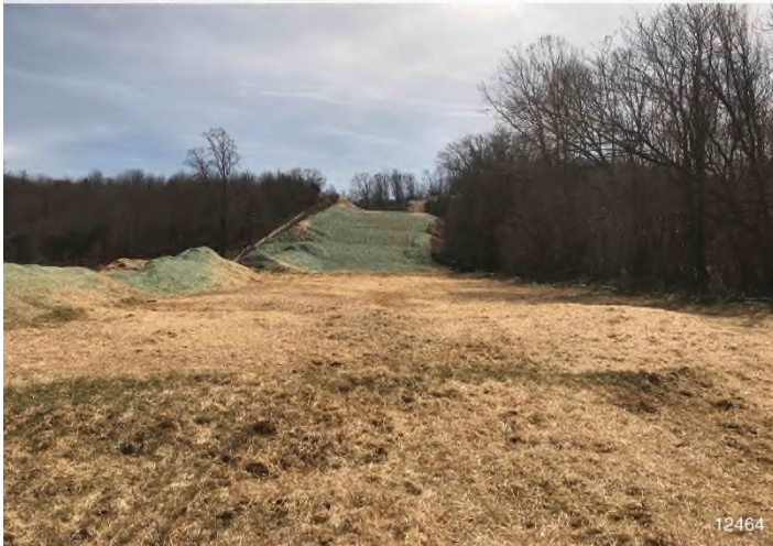
Figure 3: STA 12464+00 – Controls in place and functioning properly. Area stabilized with straw. BRG: 159°S (T) LAT: 37.228214 LON: -80.203414 ±16ft ALT: 1215ft
