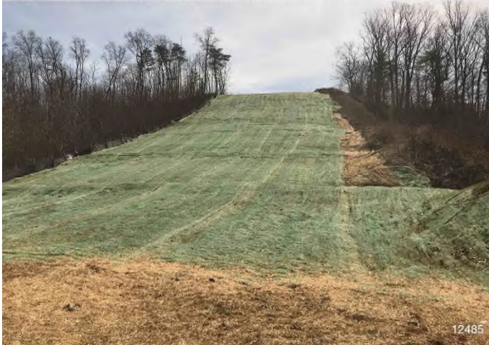
Figure 1: STA 12485+00 – Controls in place and functioning properly. Area stabilized with erosion matting. BRG: 153°SE (T) LAT: 37.223296 LON: -80.213922 ±541ft ALT: 1272ft
