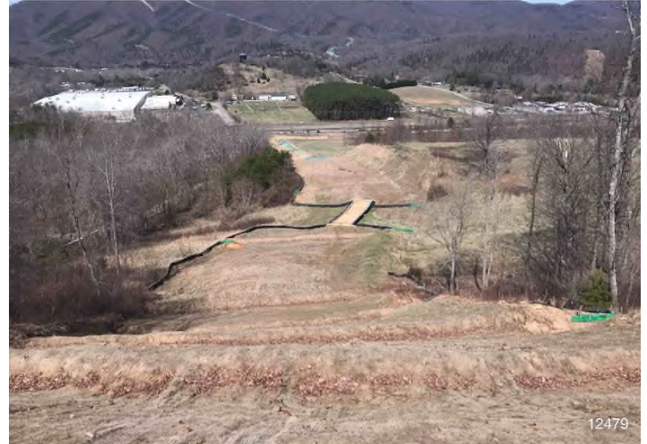
Figure 2: STA 12479+00 – Controls in place and functioning properly. Area stabilized with erosion matting. BRG: 341°N (T) LAT: 37.234050 LON: -80.204574 ±541ft ALT: 1258ft
