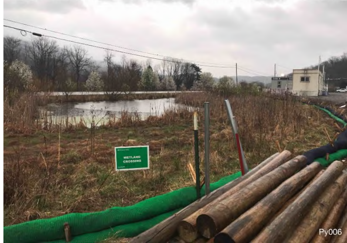
Figure 1: Pipe Yard 006 – Controls in place and functioning properly. BRG: 62°NE (T) LAT: 37.235693 LON: -80.228588 ±98ft ALT: 1350ft
