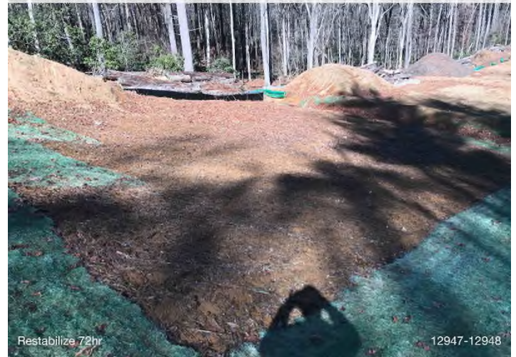
Figure 2: STA 12947+00 to 12948+00 – Re-stabilization needed. BRG: 300°NW (T) LAT: 37.136997 LON: -80.138890 ±16ft ALT: 2677ft
