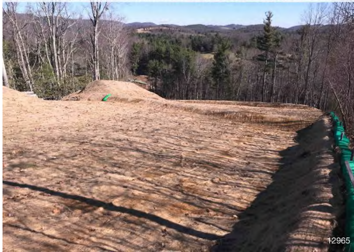
Figure 1: STA 12965+00 – Controls in place and functioning properly. Area stabilized with erosion matting. BRG: 12°N (T) LAT: 37.124623 LON: -80.142293 ±17962ft ALT: 2701ft
