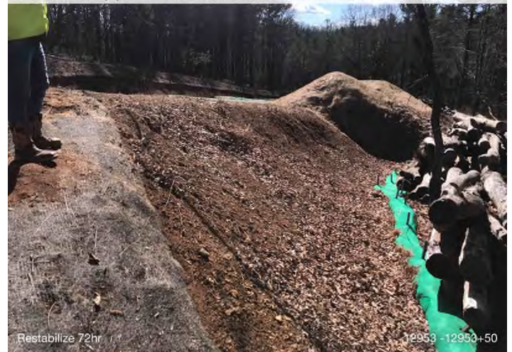
Figure 4: STA 12953+00 to 12953+50 – Re-stabilization needed.
