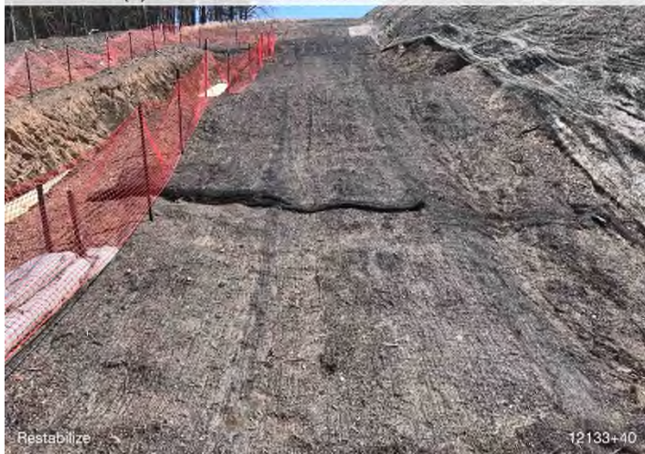
Figure 3: STA 12144+50 to 12145+00 – Re-stabilization needed.
