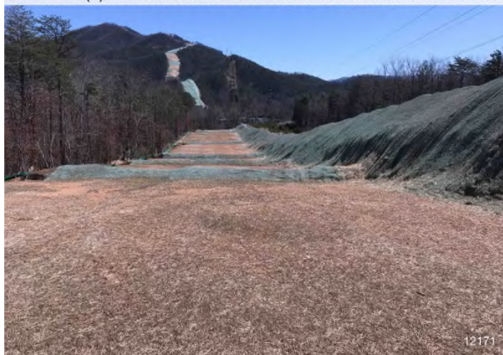
Figure 4: STA 12171+00 – Controls in place and functioning properly. Area stabilized with straw.
