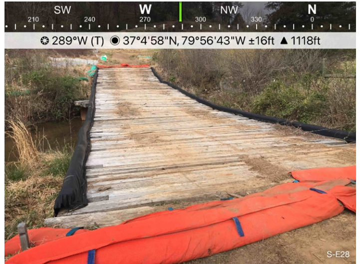
Figure 4: Designated crossing W-E7, ECD's are in place.
