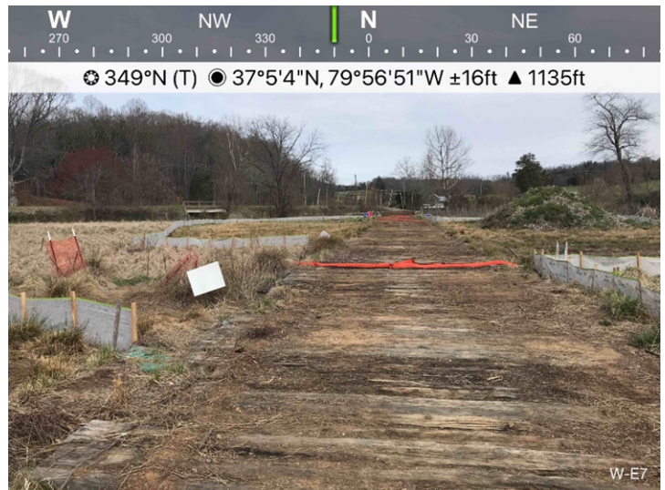
Figure 4: Designated crossing W-E7, ECD's are in place.
