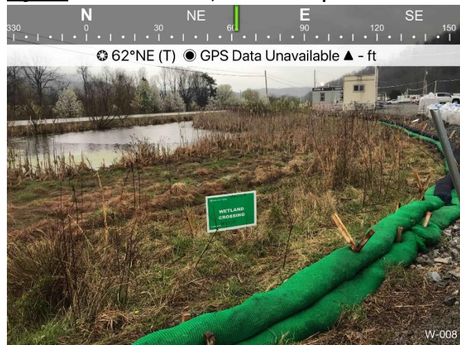
Figure 2: Resource W-008, ECD's are in place.
