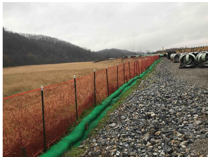
Figure 4: Laydown yard 49, ECD's are in place.
