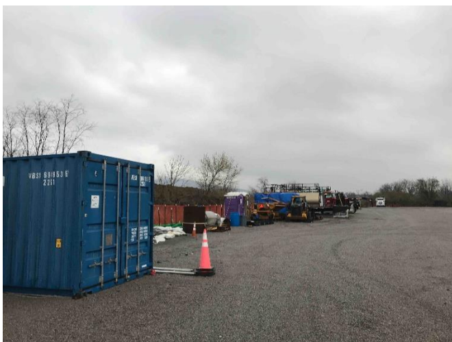
Figure 3: Laydown yard 49: covered storage, protected sanitary waste, and perimeter controls in place.
