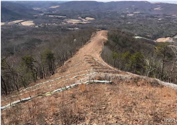
Figure 3: STA 12253+00 – Controls in place and functioning properly.
