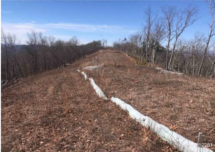
Figure 3: STA 12253+00 – Controls in place and functioning properly.
