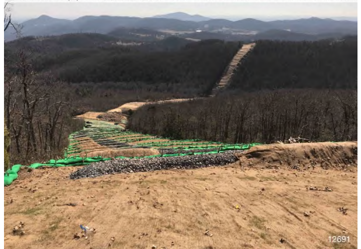
Figure 4: STA 12691+00 – Controls in place and functioning properly. Area stabilized with erosion matting.
