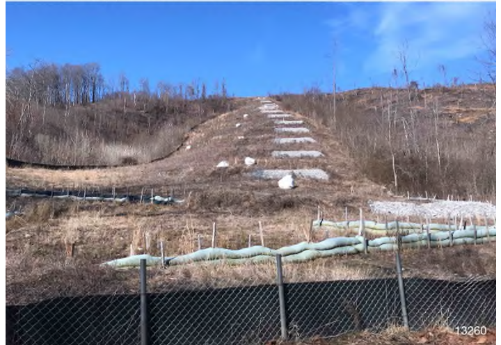
Figure 4: STA 12691+00 – Controls in place and functioning properly. Area stabilized with erosion matting.
