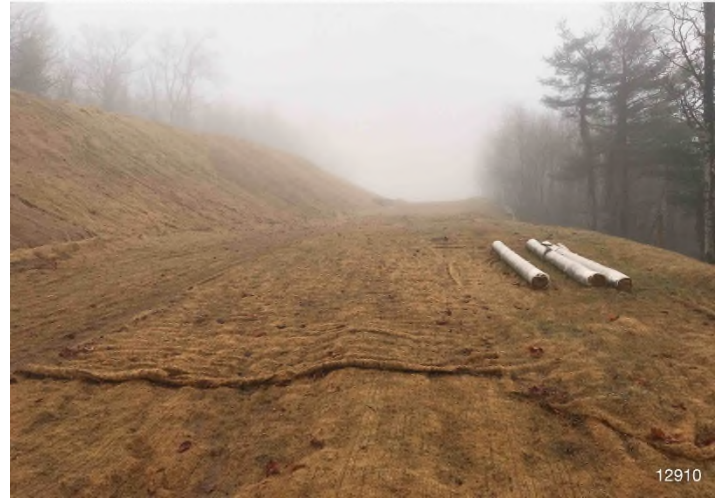
Figure 2: STA 12910+00 – Controls in place and functioning properly. Area stabilized with erosion matting. BRG: 85°E (T) LAT: 37.119516 LON: -80.137216 ±21305ft ALT: 2686ft
