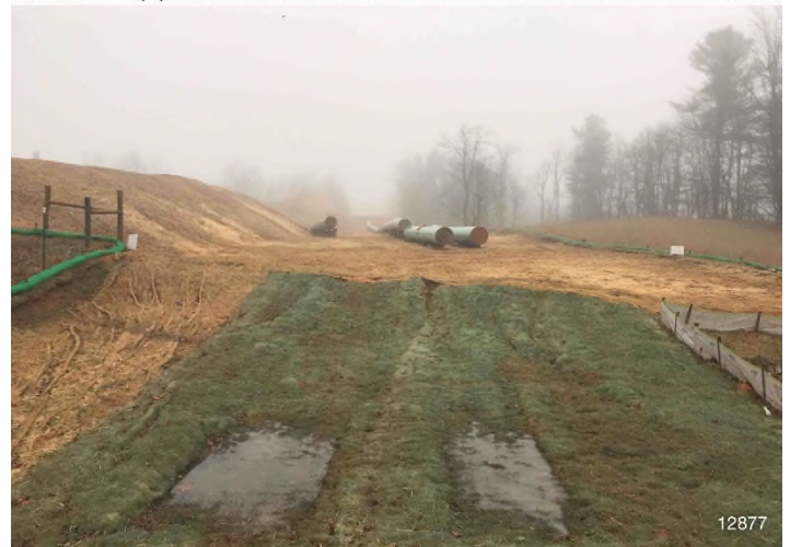
Figure 4: STA 12877+00 – Controls in place and functioning properly. Area stabilized with erosion matting and straw. BRG: 17°N (T) LAT: 37.154295 LON: -80.125023 ±7391ft ALT: 2617ft
