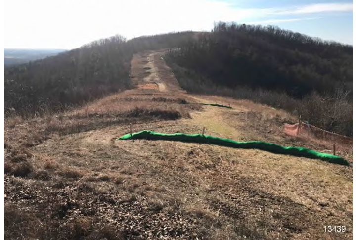
Figure 2: STA 13439+00 – Controls in place and functioning properly.
