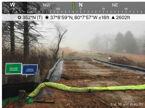
Figure 3: Designated crossing S-KL55 & W-KL51, ESC's are in place and functioning.
