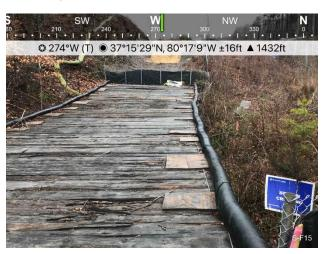
Figure 4: St12233+23, ECD's are in place and functioning.
