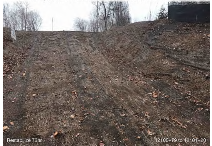
Figure 4: STA 12100+70 to 12101+20 – Re-stabilization needed. Erosion control matting deteriorated.
