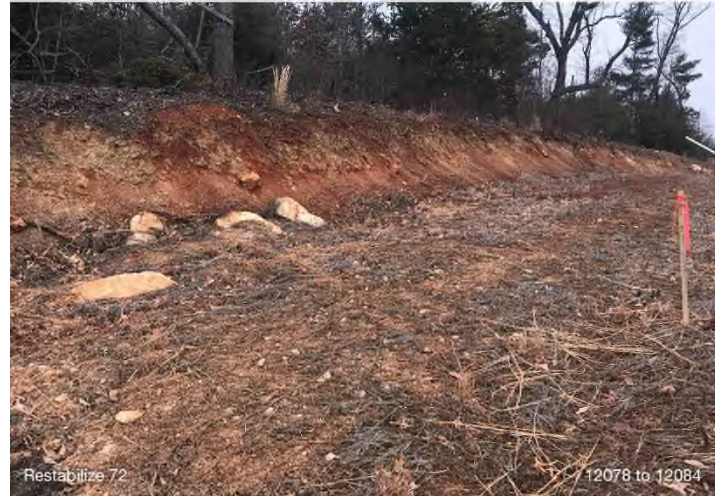
Figure 4: STA 12100+70 to 12101+20 – Re-stabilization needed. Erosion control matting deteriorated.
