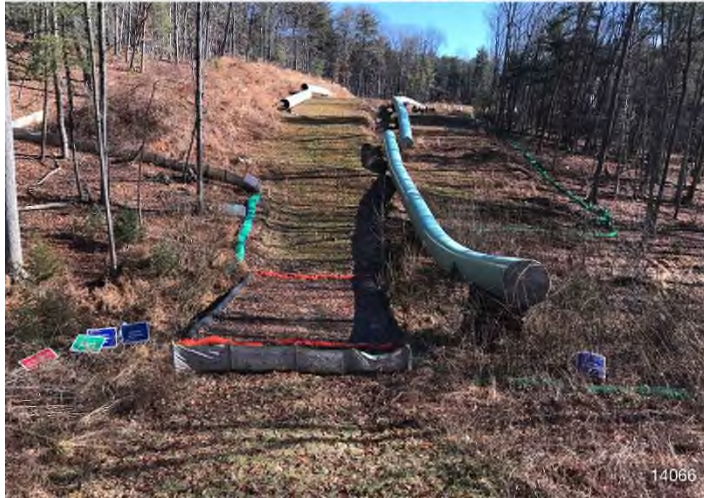
Figure 3: STA 14112+00 – Controls in place and functioning properly.
