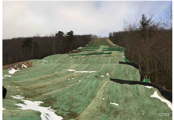
Figure 4: STA 12703+00 – Controls in place and functioning properly. BRG: 294°NW (T) LAT: 37.191014 LON: -80.153724 ±32ft ALT: 3396ft
