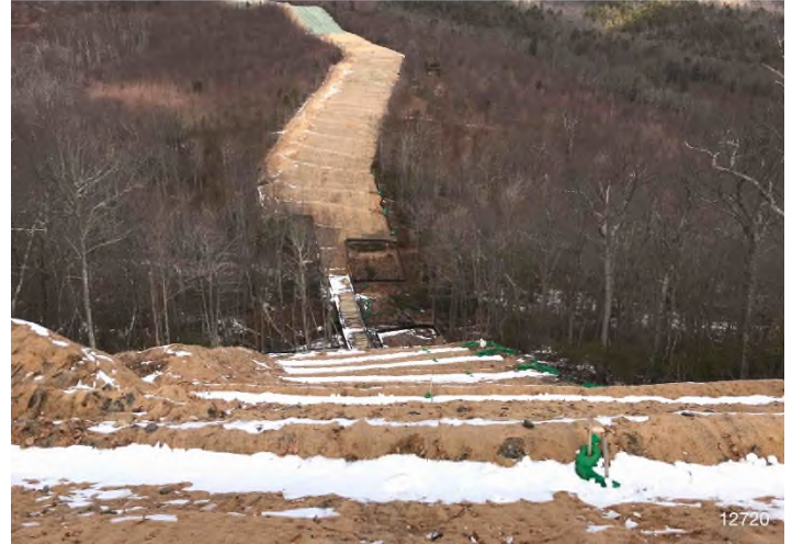
Figure 2: STA 12720+00 – Controls in place and functioning properly. BRG: 350°N (T) LAT: 37.186471 LON: -80.150607 ±164ft ALT: 3262ft
