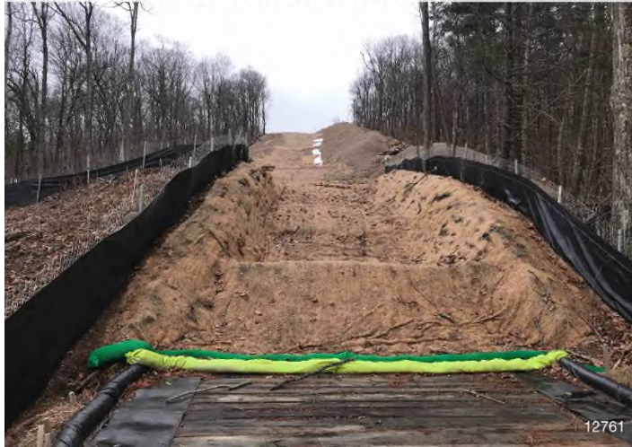
Figure 1: STA 12761+00 – Controls in place and functioning properly. Area stabilized with erosion matting. BRG: 147°SE (T) LAT: 37.179111 LON: -80.141374 ±164ft ALT: 2904ft
