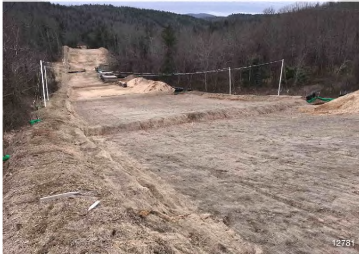
Figure 3: STA 12781+00 – Controls in place and functioning properly. Area stabilized with erosion matting. BRG: 179°S (T) LAT: 37.178437 LON: -80.135868 ±6614ft ALT: 2870ft
