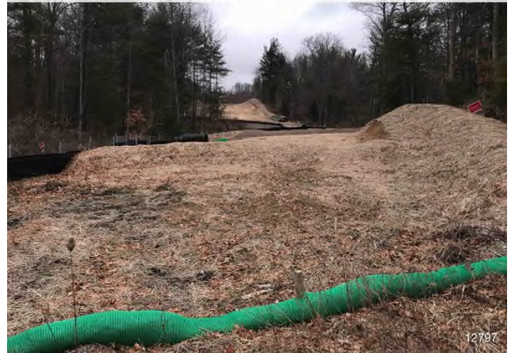
Figure 4: STA 12797+00 – Controls in place and functioning properly. BRG: 21°N (T) LAT: 37.178961 LON: -80.134189 ±6040ft ALT: 2717ft
