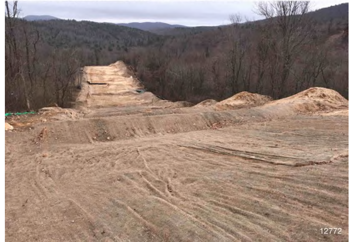
Figure 2: STA 12772+00 – Controls in place and functioning properly. Area stabilized with erosion matting. BRG: 193°S (T) LAT: 37.181551 LON: -80.133599 ±6896ft ALT: 2981ft
